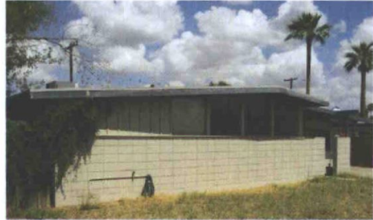
One of the most intact of the Town and Country residences, this house features simple but Attractive concrete block at the base, board and batten on the upper wall, the original window band and the original open entrance.
