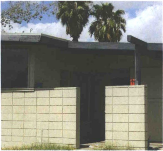
This entry is in original form, including the exposed rafter that was intended to be both ornamental and structural.
