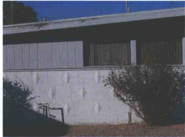
The vertical wood siding on the upper half on the front façade should be maintained.
