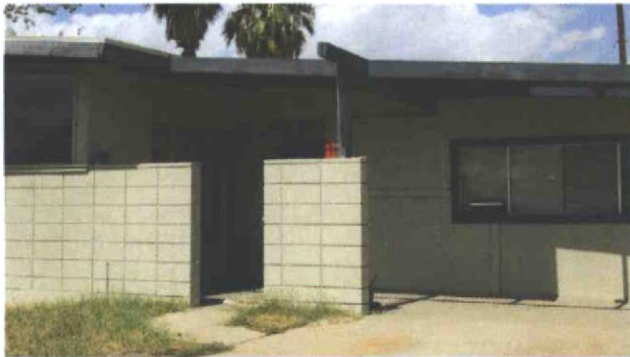
This carport was successfully enclosed to expand the interior space without altering the overall design of the house. The wall was set back beneath the roof form, and the sense of "openness" at the entry was retained.
