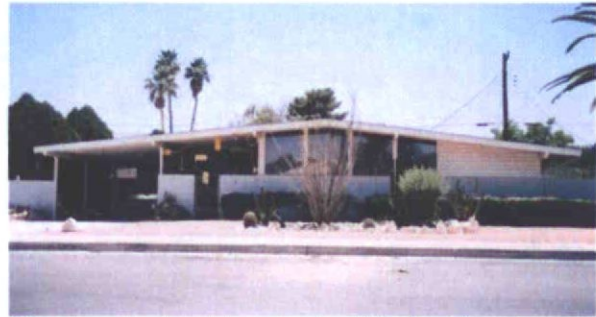
The strong horizontal emphasis of the front façade should be maintained. Avoid changes to the basic shape and massing of the home such as placing something on the roof.
