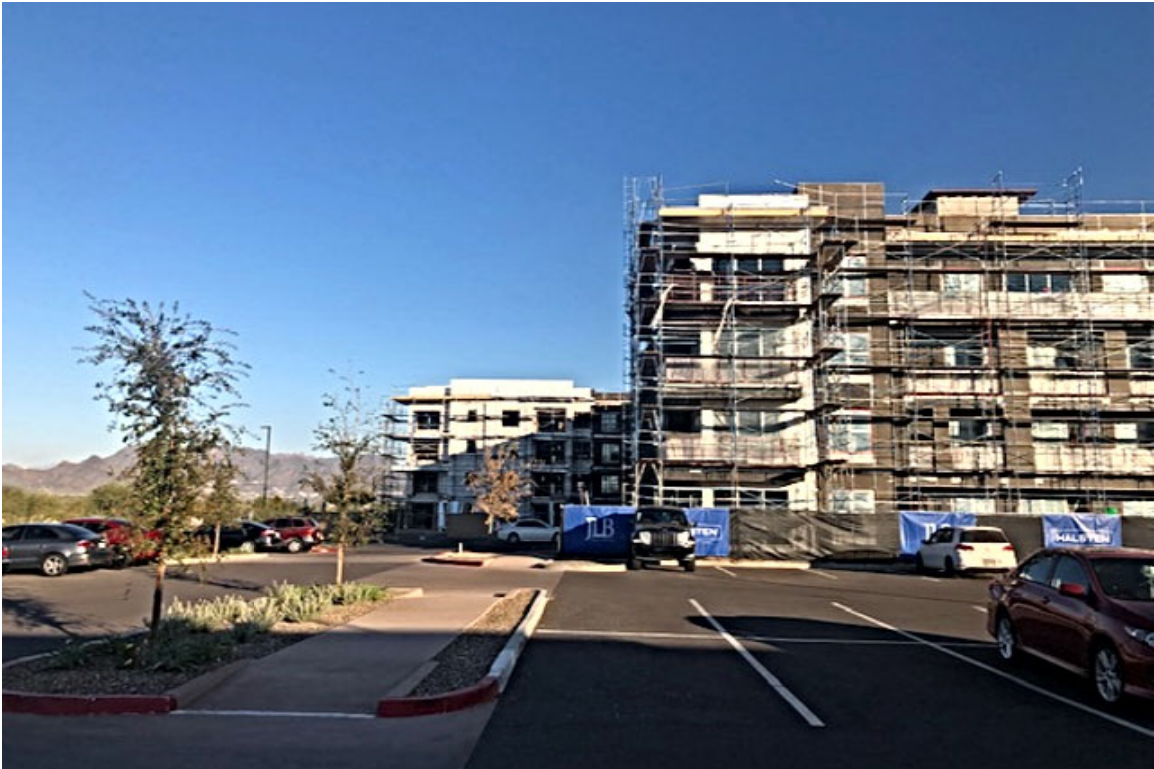
West elevation, north end
