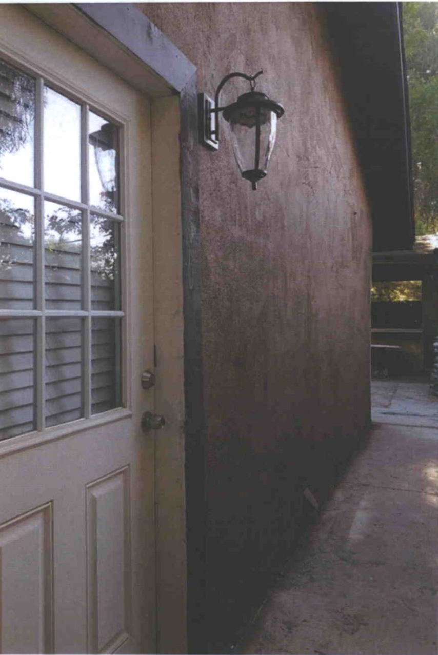
Project Variance Request Area (Citation Area) South Elevation – Looking East)
