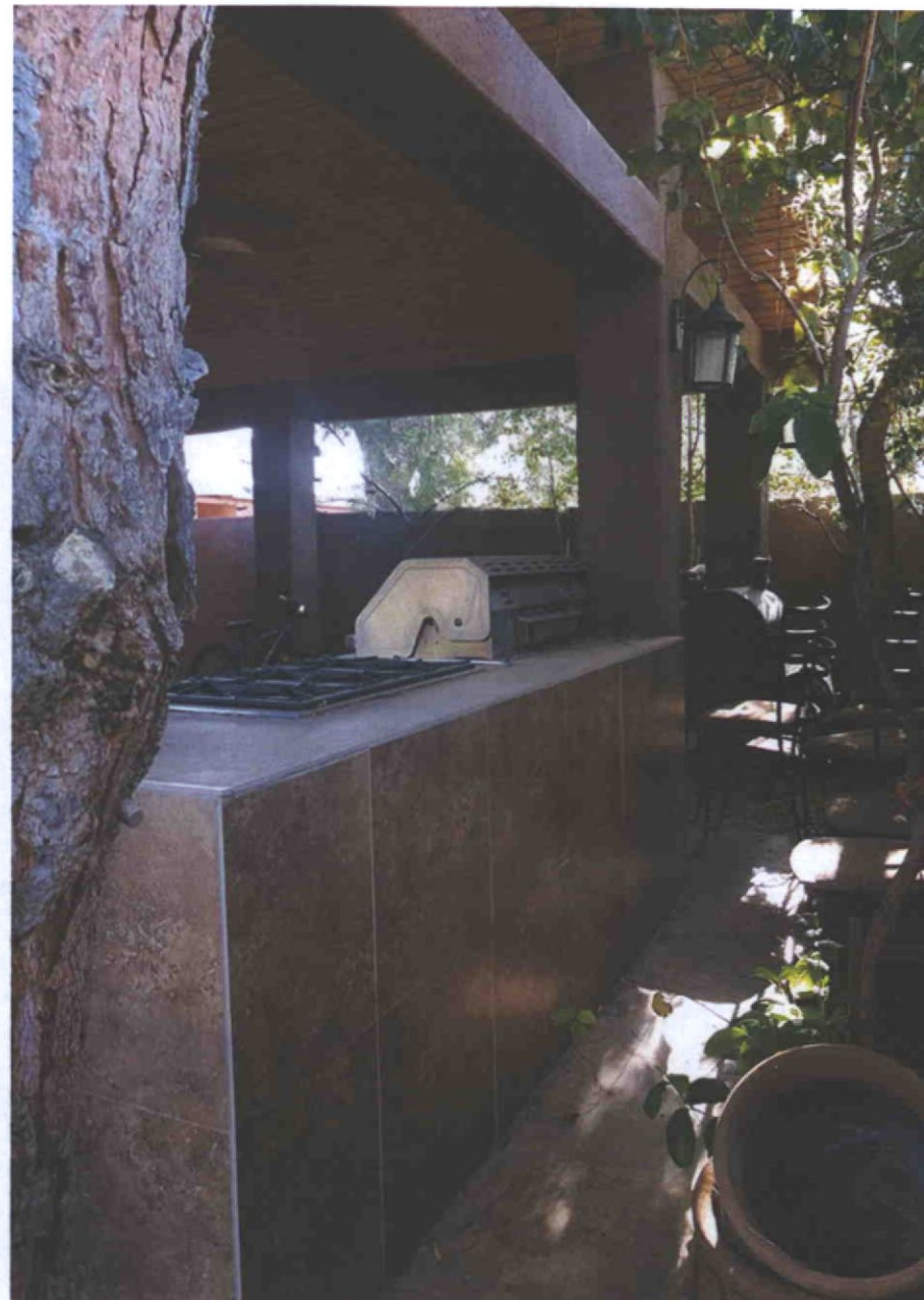
Other Unpermitted Addition Area (South Elevation – Looking East)
