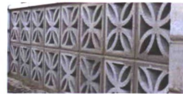
'W2' BREEZE WALL Manufacturer: Superlite Block Product: EL DORADO Color: NATURAL GREY
