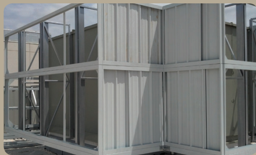
Installation of screen around unit with pipe-chase.
