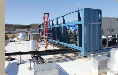
Screen being installed to avoid existing roof piping.
