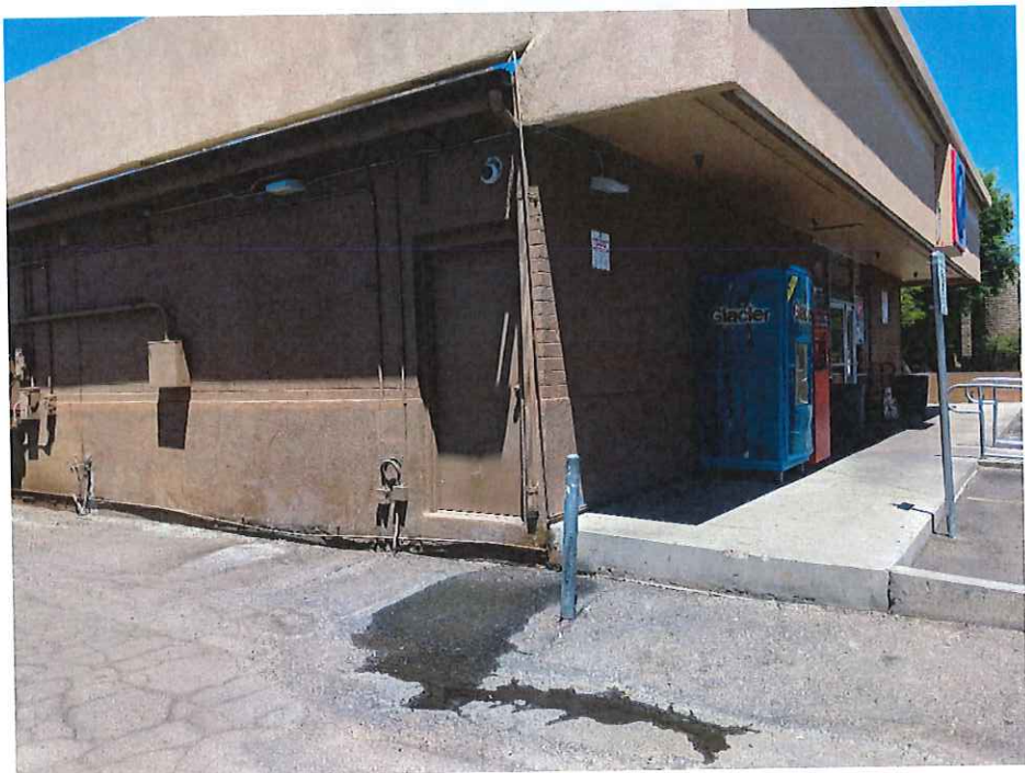
2. NE corner looking NW
