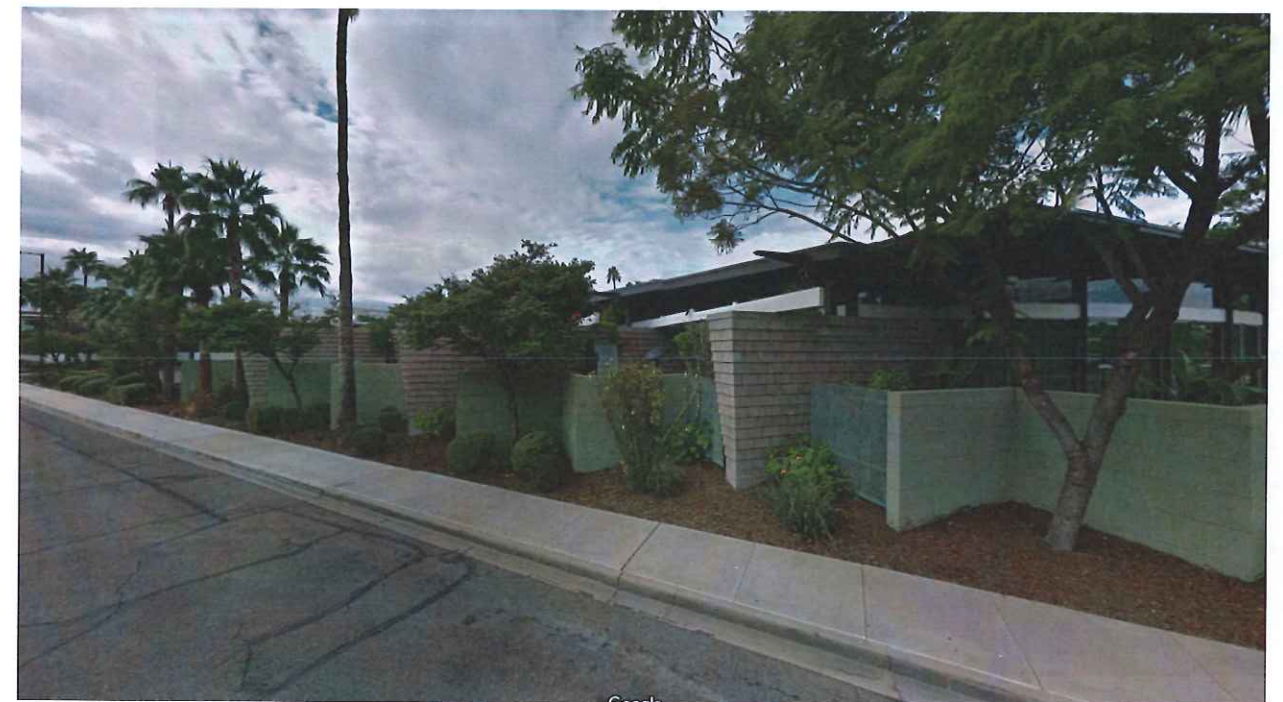
8 NW corner looking SW
