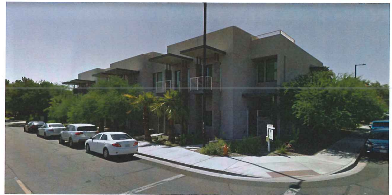
15 SW corner looking SE
