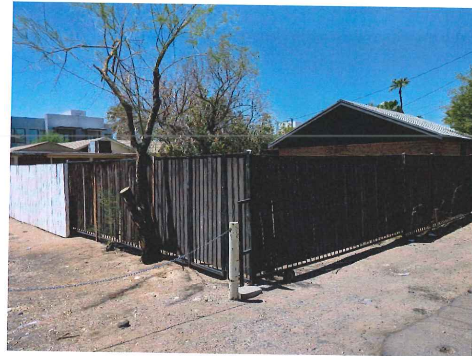
3. NE corner looking SW
