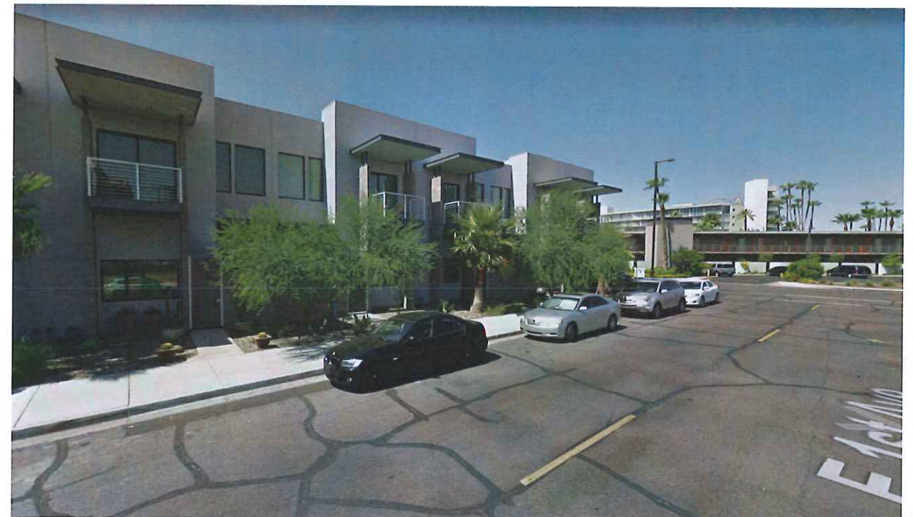
12 SE corner looking SW
