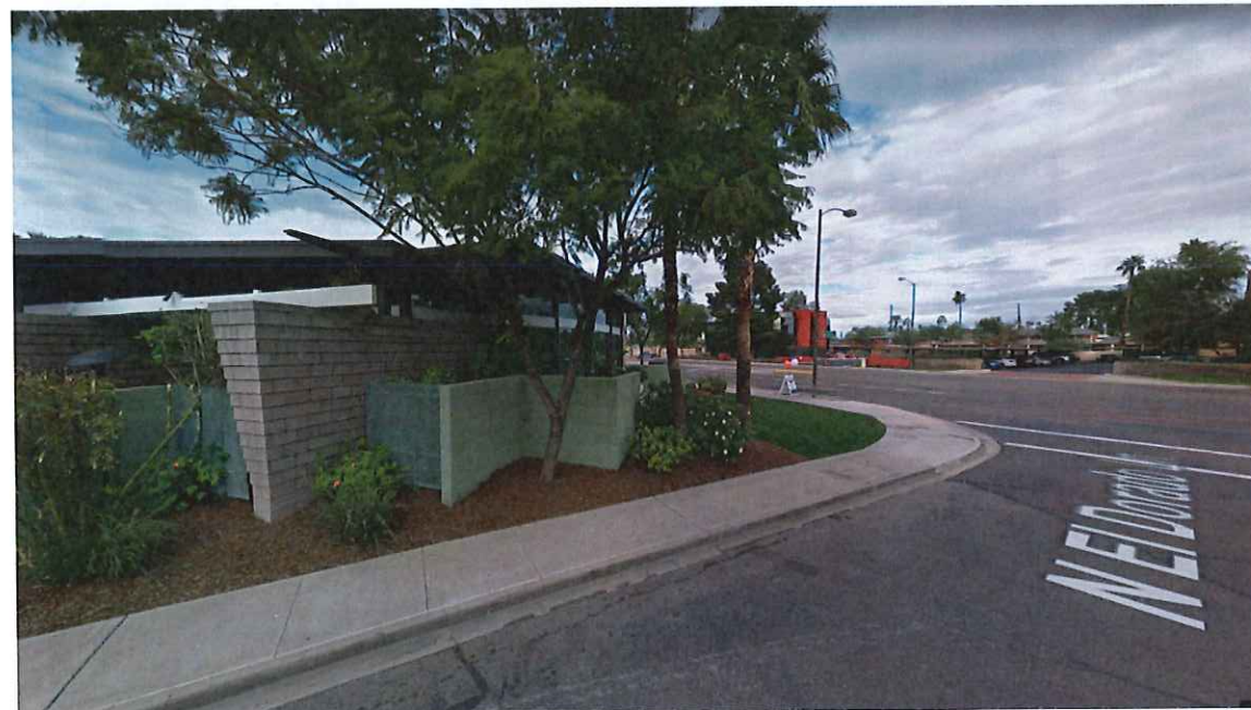
6. NW corner looking NW
