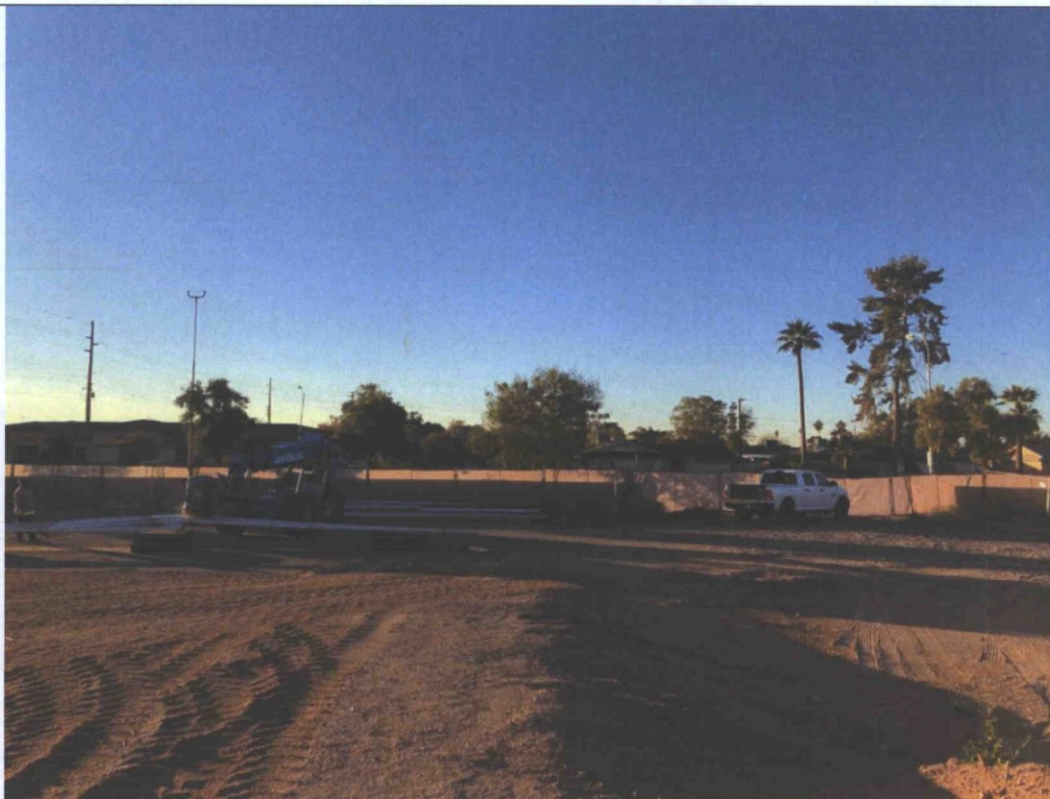
PHOTO #16 – View to South
