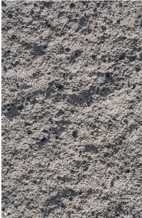
W1, W2 - Split Face CMU Shown for texture only. See paint samples for color.
