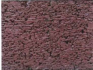
SMOOTH FACE INTEGRAL COLOR CMU BLOCK HORIZ. RAKED JOINT, VERT. FLUSH JOINT SUPERLITE PURPLE HART
