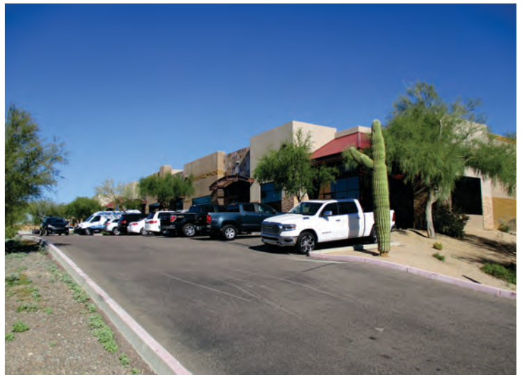
Photo 15 - View of the east adjoining office/retail building, looking northeast across its driveway.
