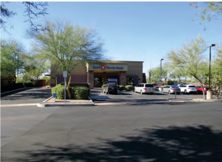
Photo 17 - View of the south adjoining BMO Harris Bank branch office, looking west across its driveway.
