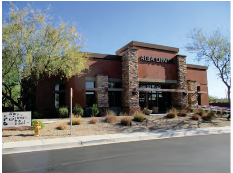
Photo 16 - View of the southeast adjoining Alba Dental building, looking east across its driveway.
