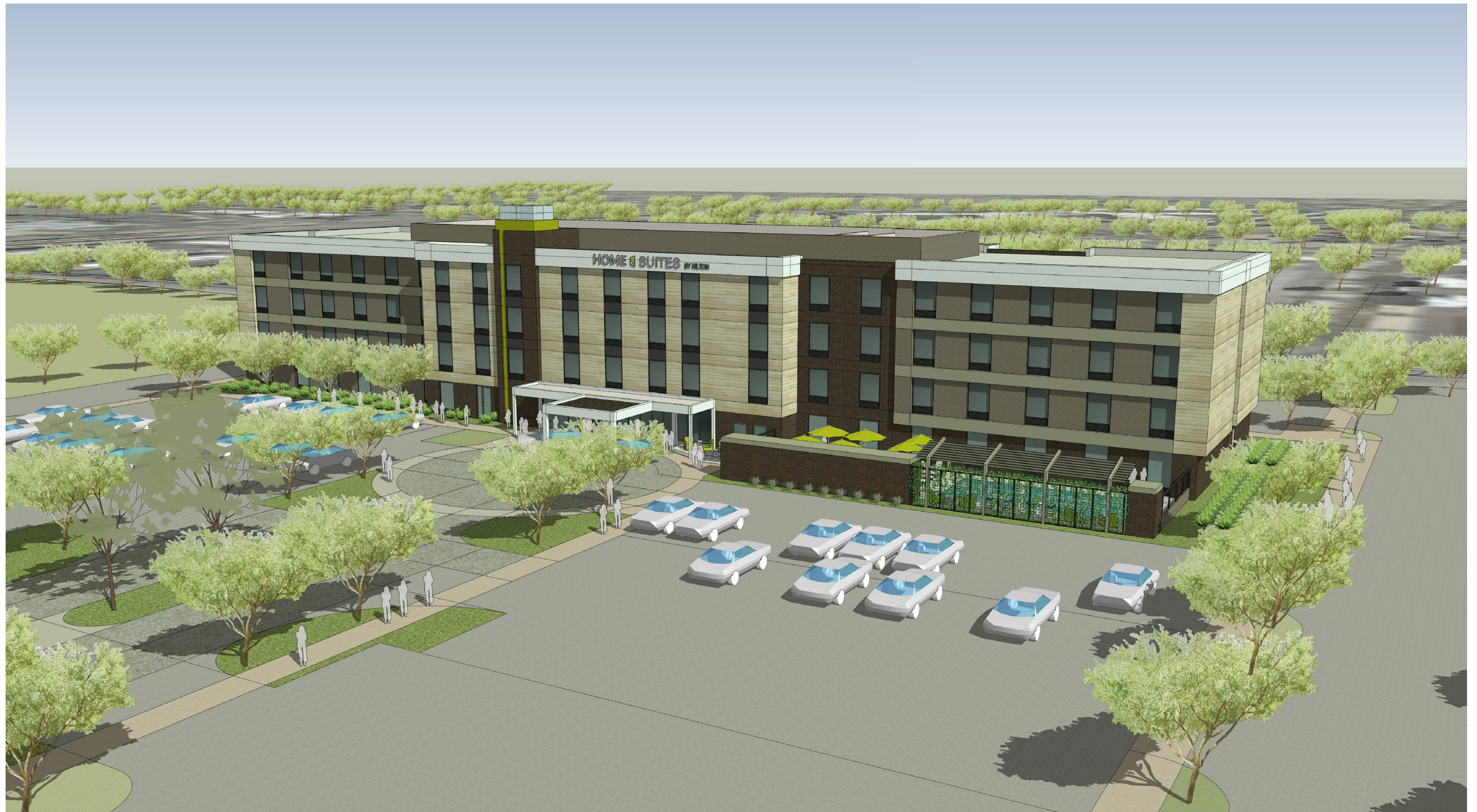
View from Southwest
