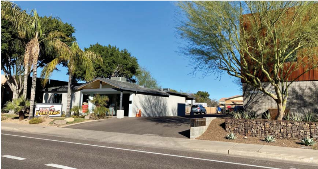
Site Photo 1: Facing Northwest from Osborn Road
