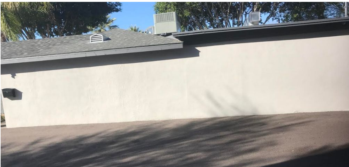
Site Photo 3: Facing West from Driveway
