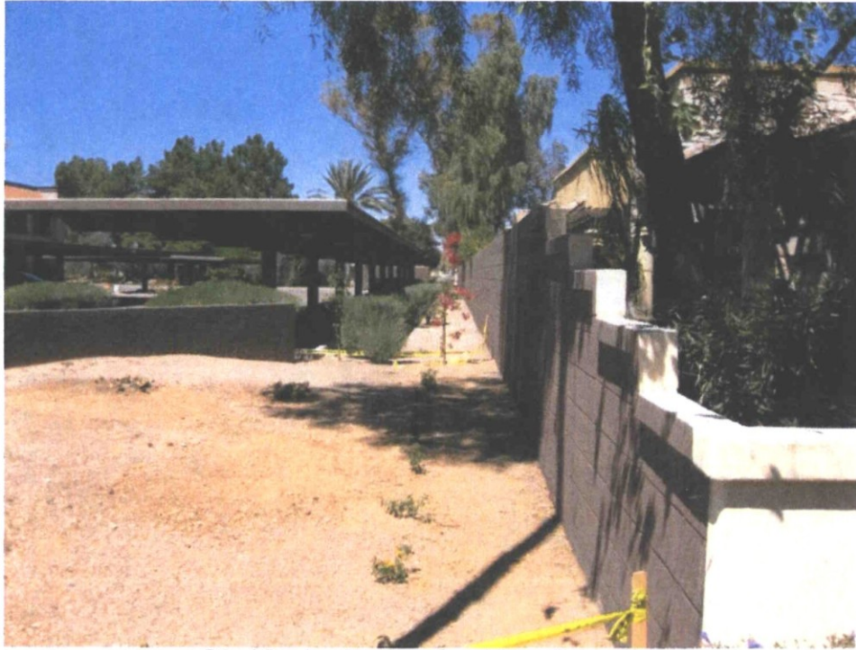
C1 - Viewing North at San Victor Drive.JPG
