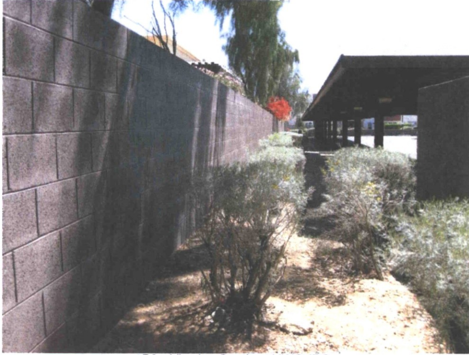
B3 - Viewing South at NWC.JPG
