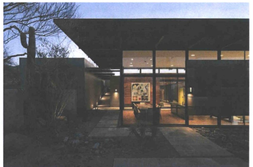
clarity of contemporary materials with protected wood soffits
