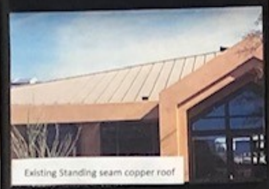
Existing Standing seam copper roof
