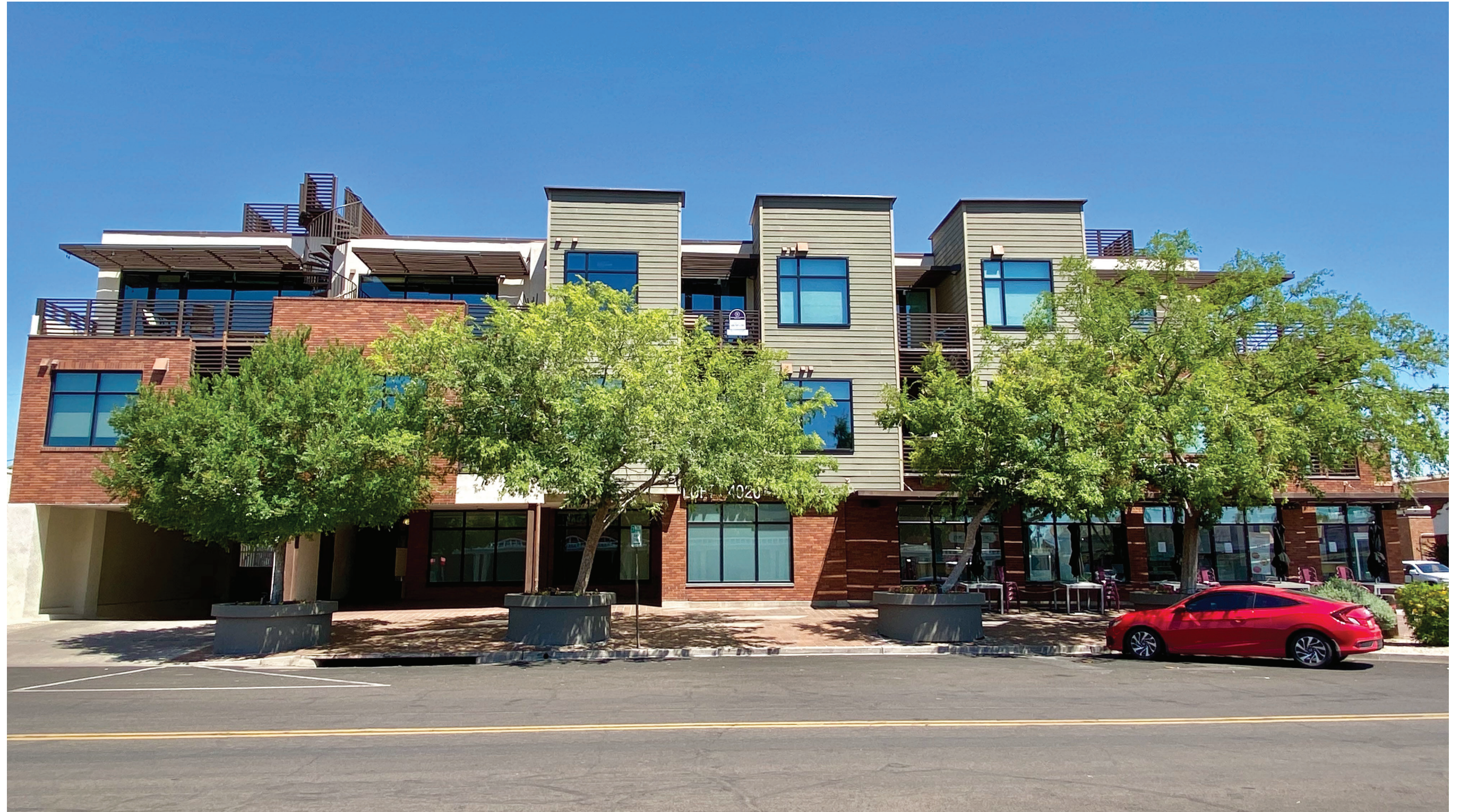
South Elevation View
