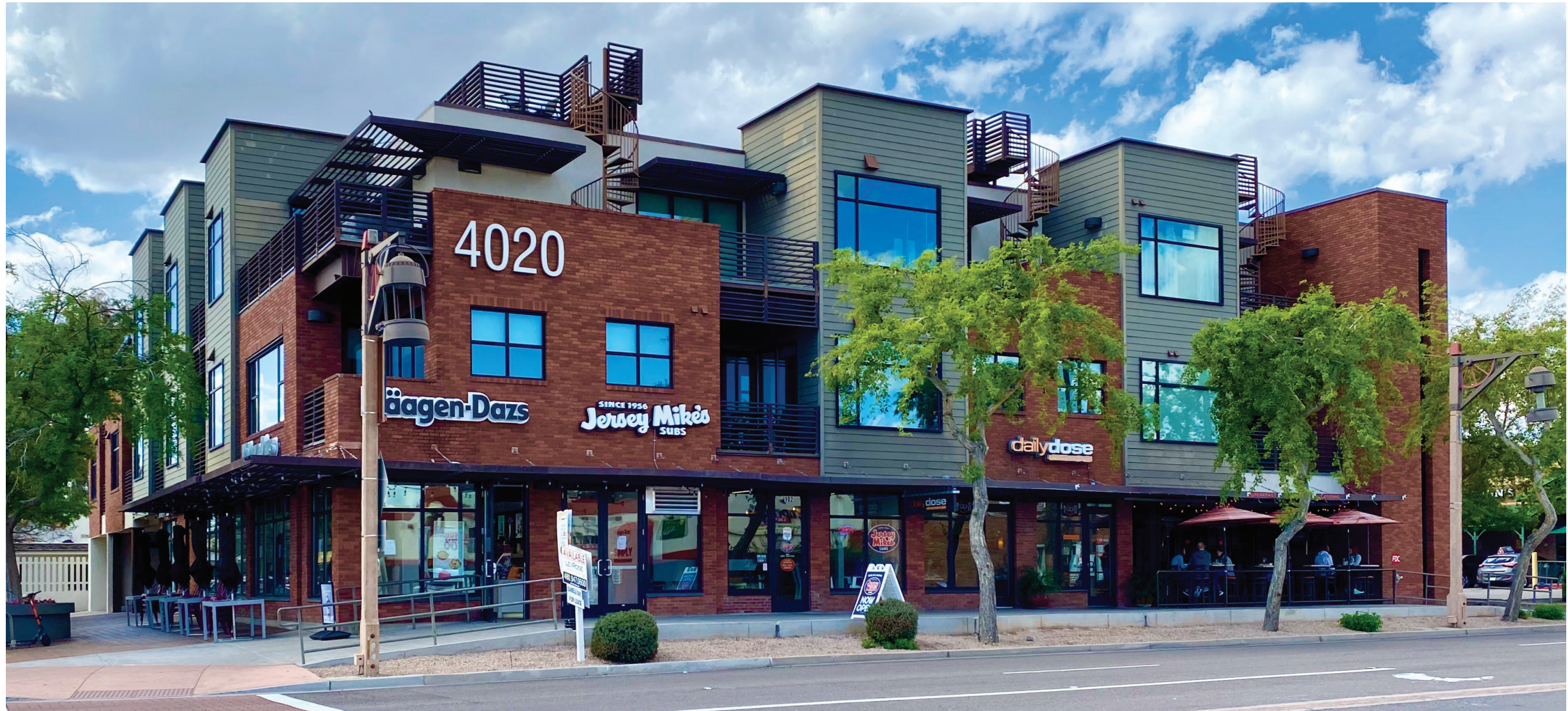
Southeast & East Elevation View
