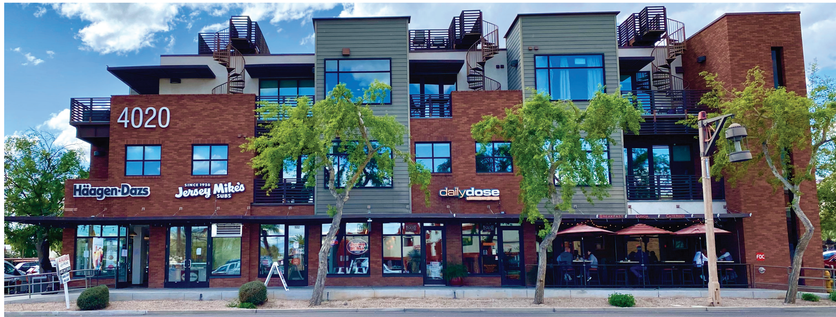
East Elevation View
