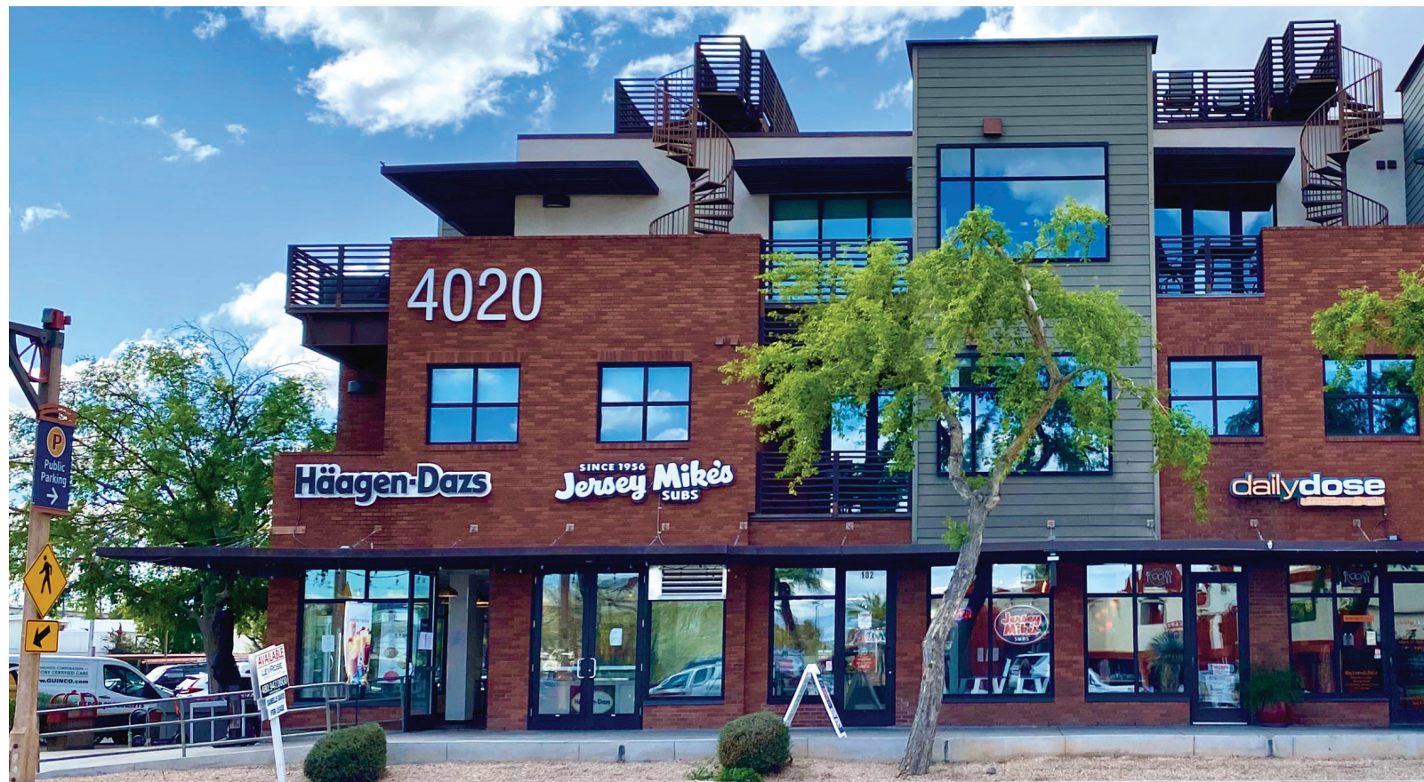
East Elevation View
