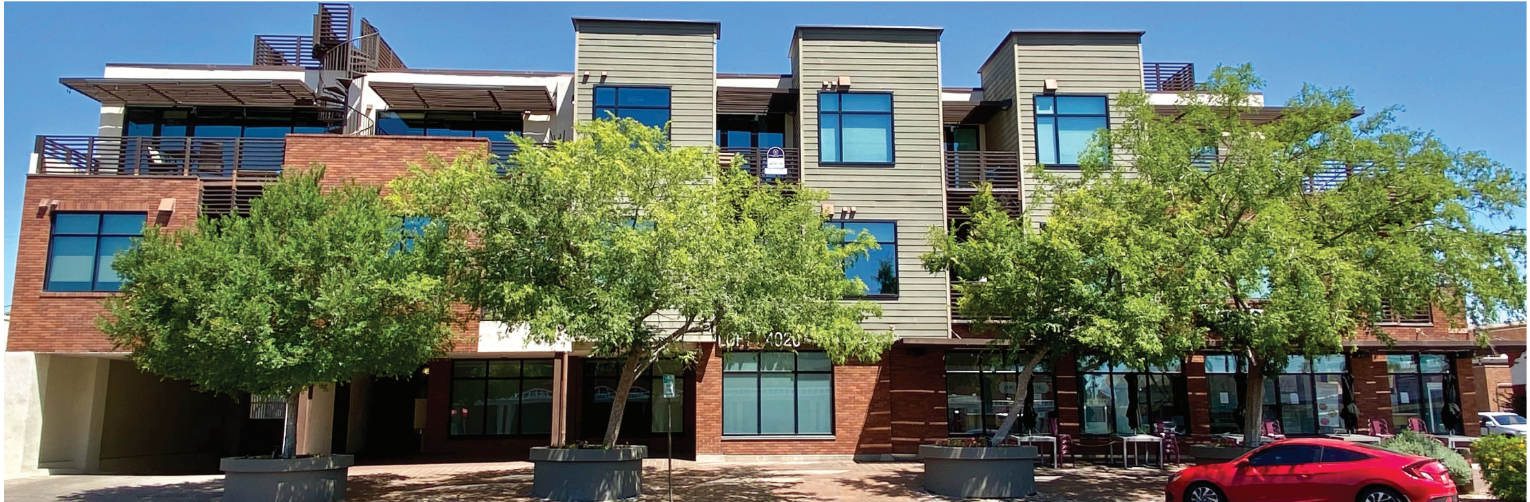
South Elevation View
