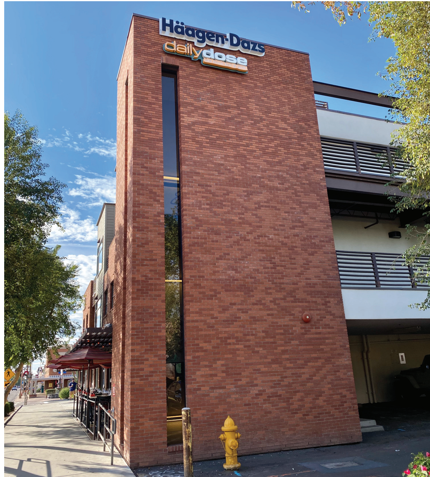
North Elevation View
