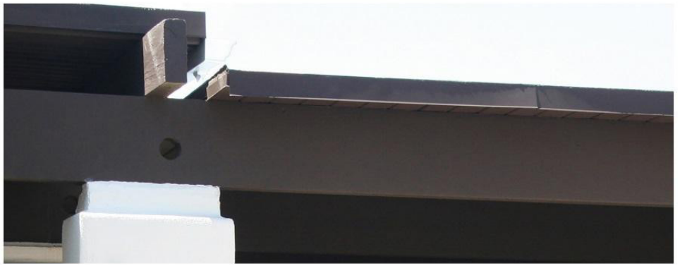
Roof extension and flashing modifications to protect exposed wood members
