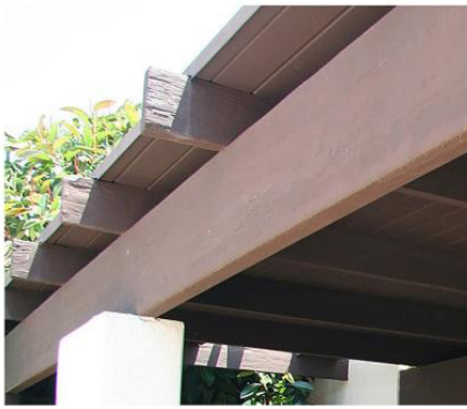
Roof extension and flashing modifications to protect exposed wood members
