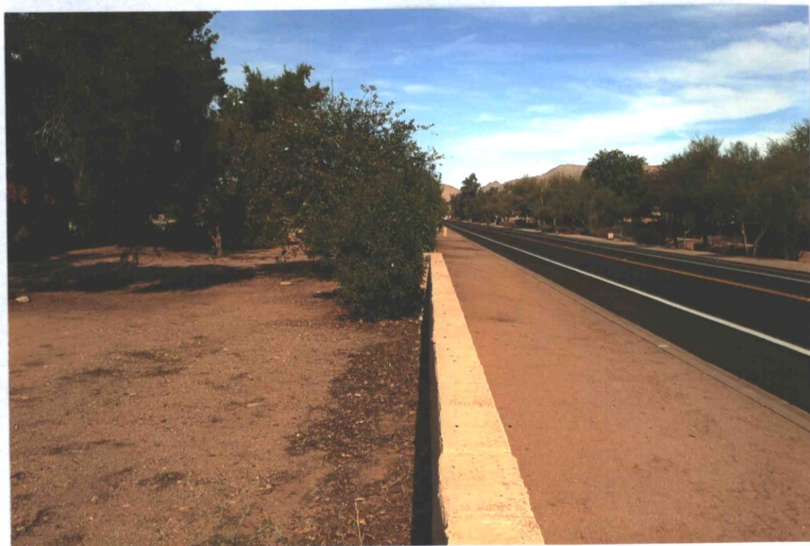
East side looking north
