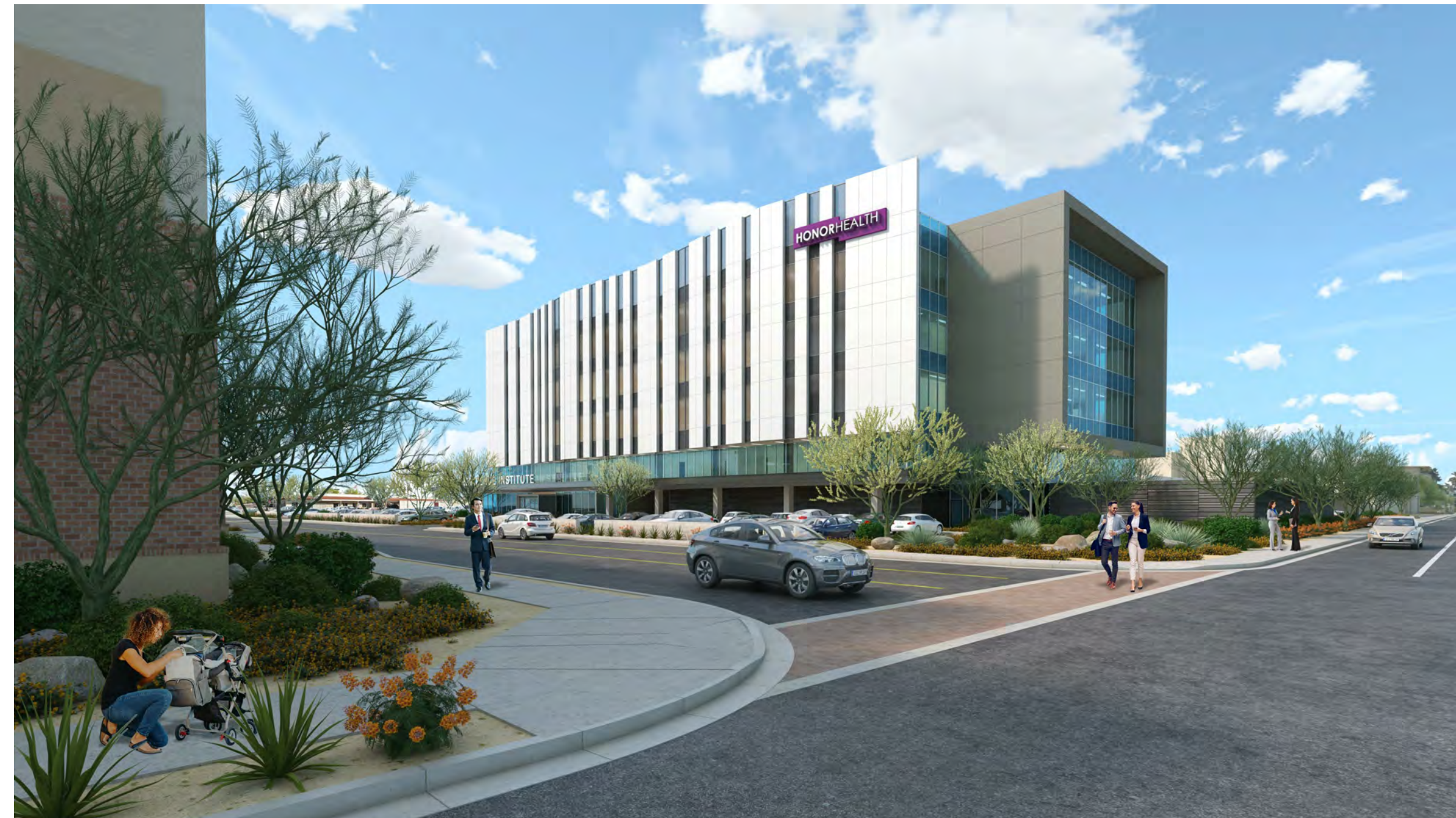
SOUTHWEST VIEW - FROM E. OSBORN ROAD
