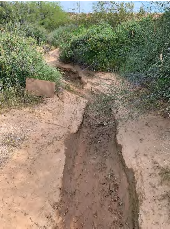
Upstream view facing northeast
