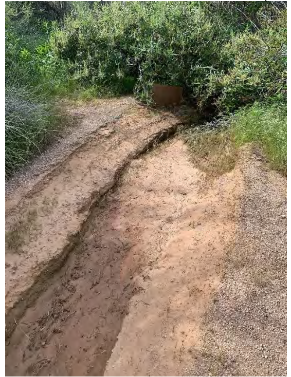
Downstream view facing southwest
