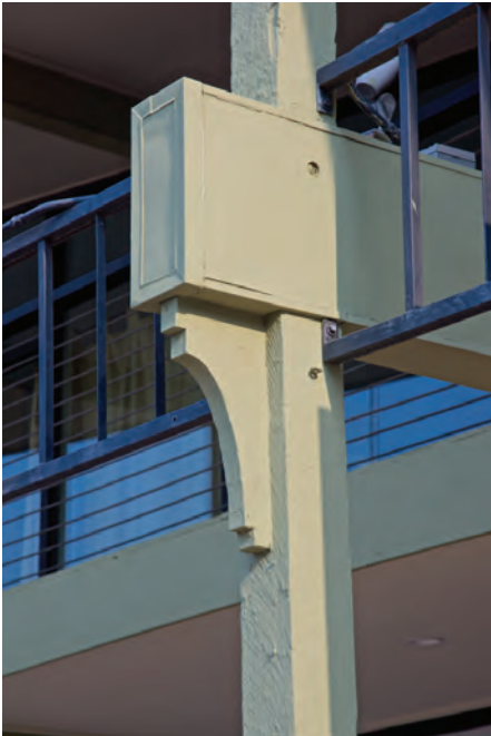
The original curved corbel design is an unusual detail for Contemporary-style beams that may be an architectural salute to the gable brackets of the earlier Kimsey farmhouse.
