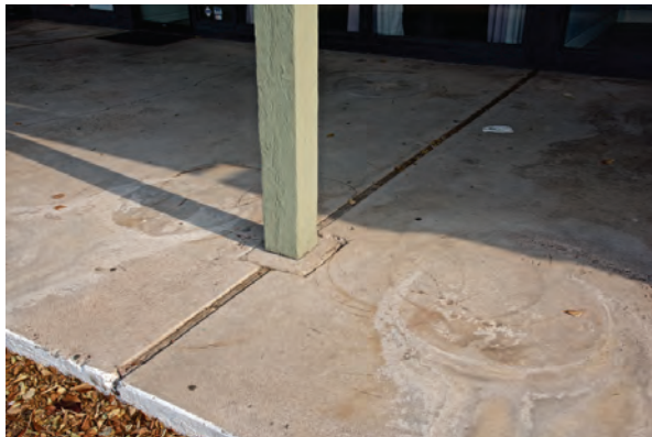
The character-defining concrete slab and redwood headers of the porch terrace have sustained staining, deterioration, and modification that affect their integrity of materials.
