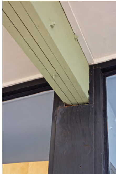
The economical laminated beams supporting the roof and second floor have been sheathed to protect from weather and to enhance their appearance.
