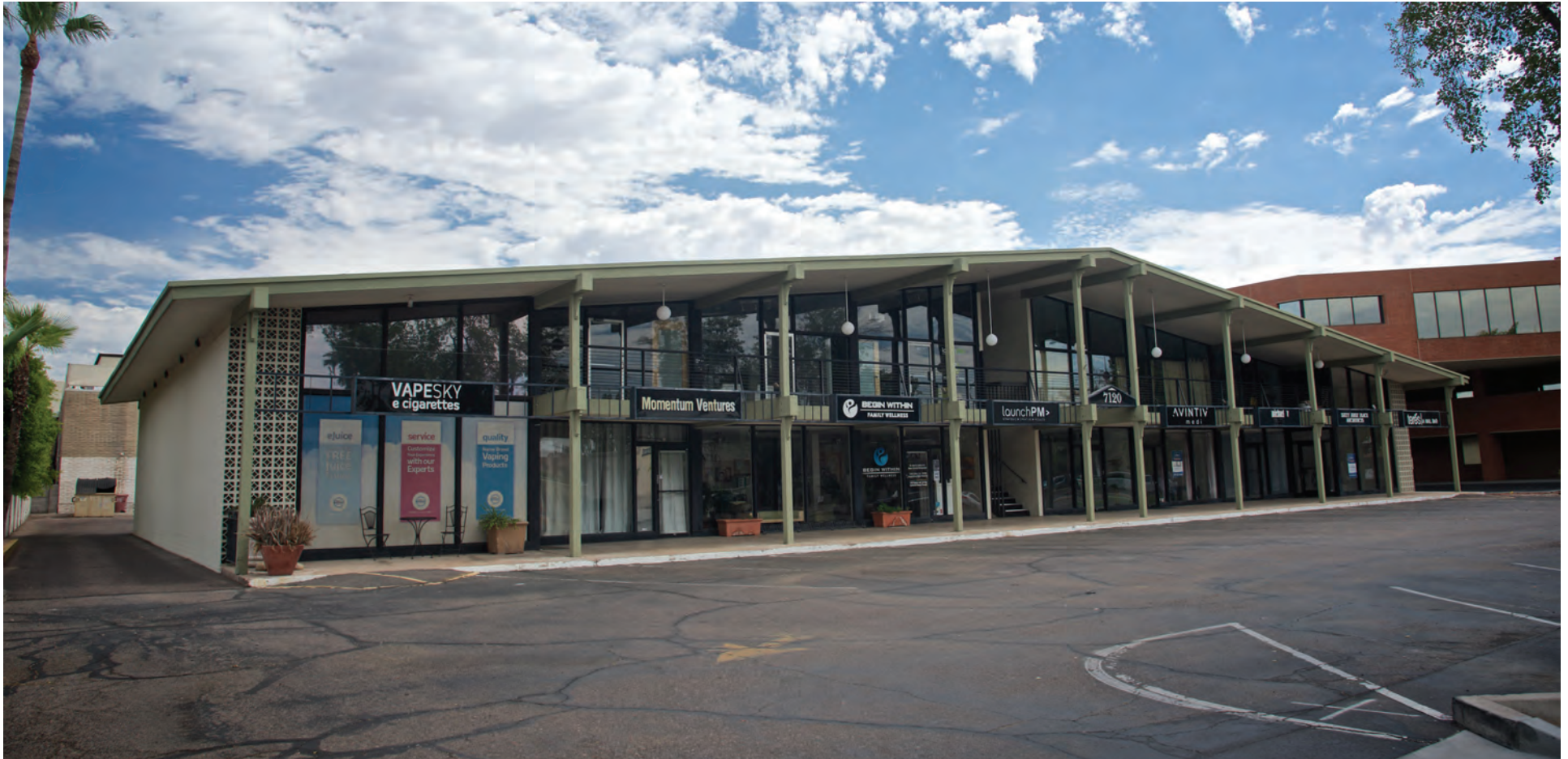
Kimsey Building front façade and parking. (August 2020)
