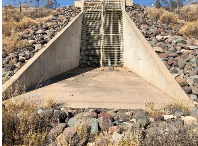
Figure 5: Dike 4 Outlet Works Photograph
