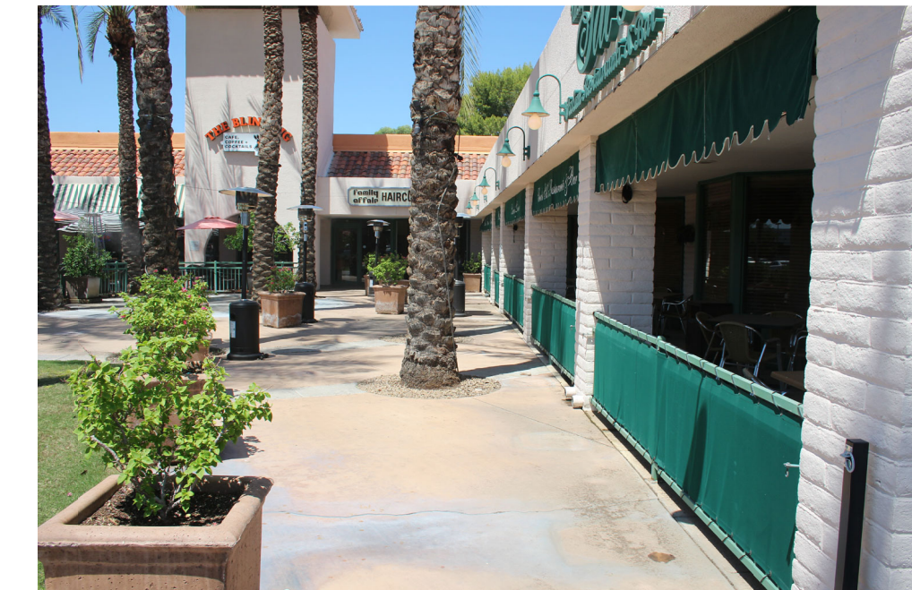
PH-01 EXISTING COURTYARD VIEW TO WEST
