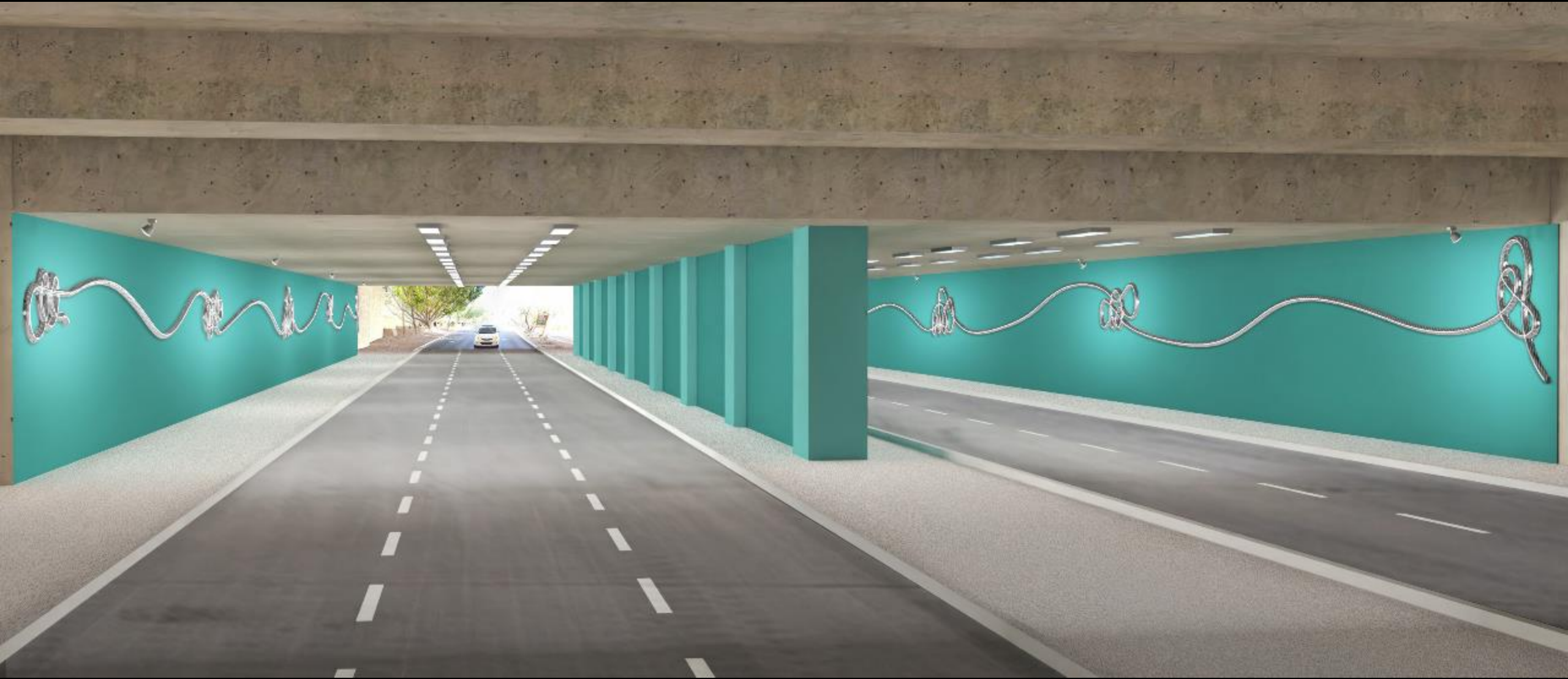
DRINKWATER BOULEVARD UNDERPASS LOOKING SOUTH OUT OF SCOTTSDALE
