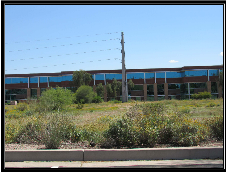
Looking south toward subject from adjacent property to north
