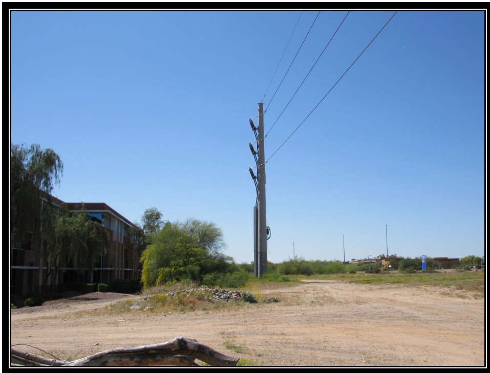
Looking west along power line easement on south side of subject
