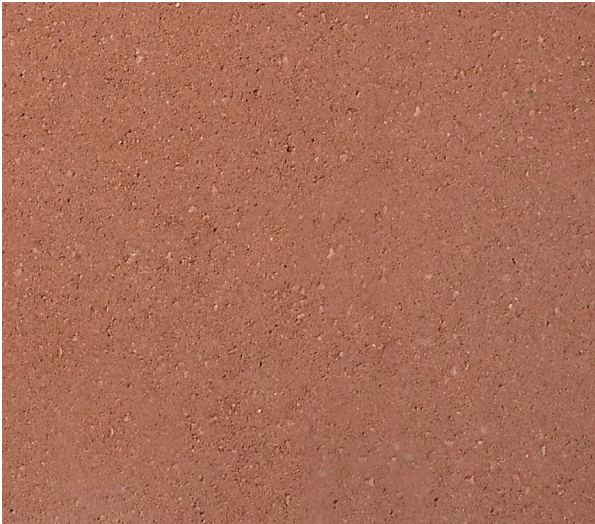
Type 2 Concrete Surfacing
