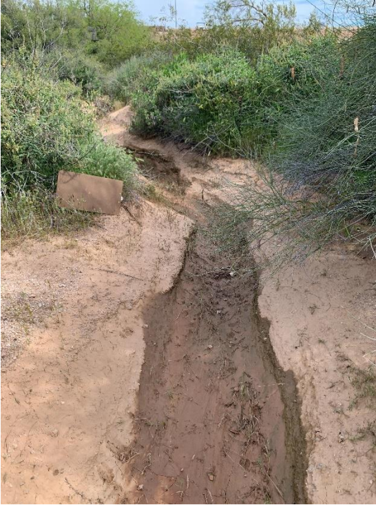
Upstream view facing northeast
