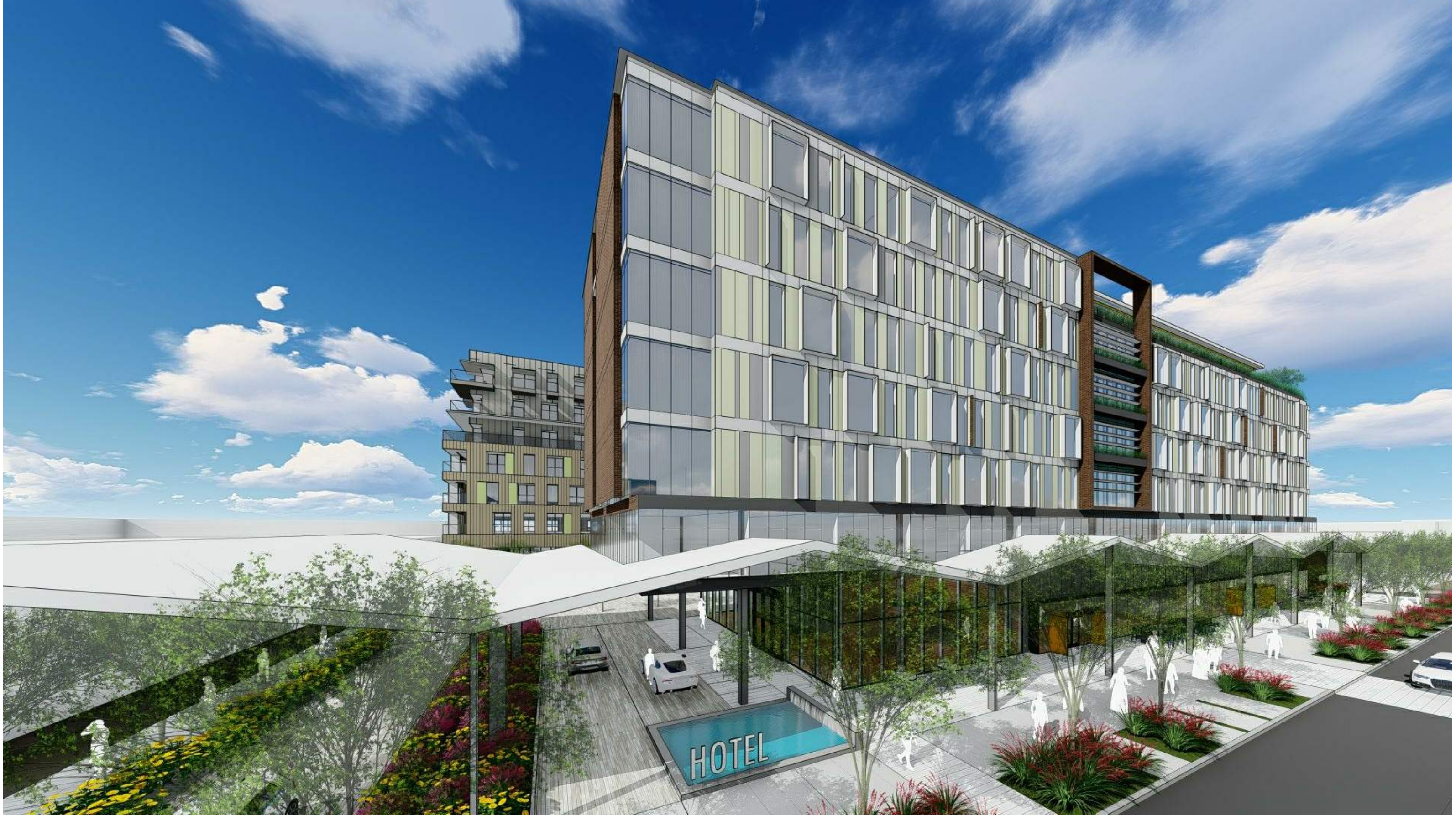
LOOKING SOUTHWEST FROM 3RD AVENUE
