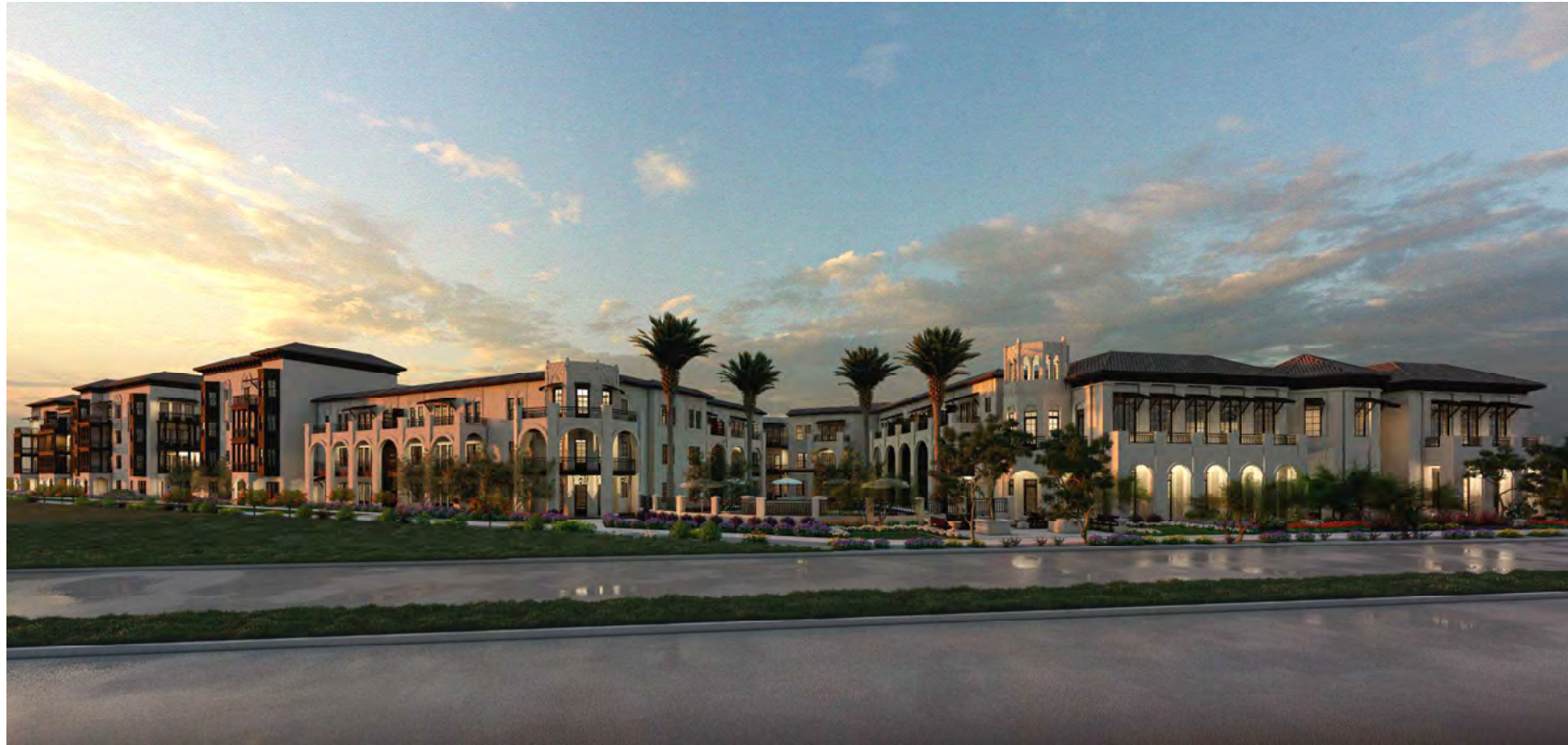
1. VIEW FROM NORTH EAST
