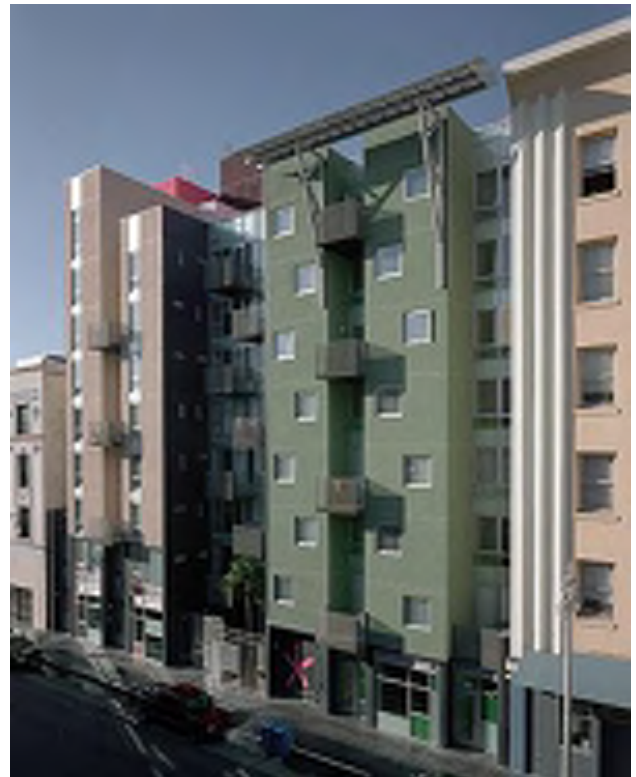
In place of parking in San Francisco, Curran House's ground floor includes community spaces, a peaceful courtyard, office space for the building developer, and additional affordable family-sized units. (Brian Rose)
