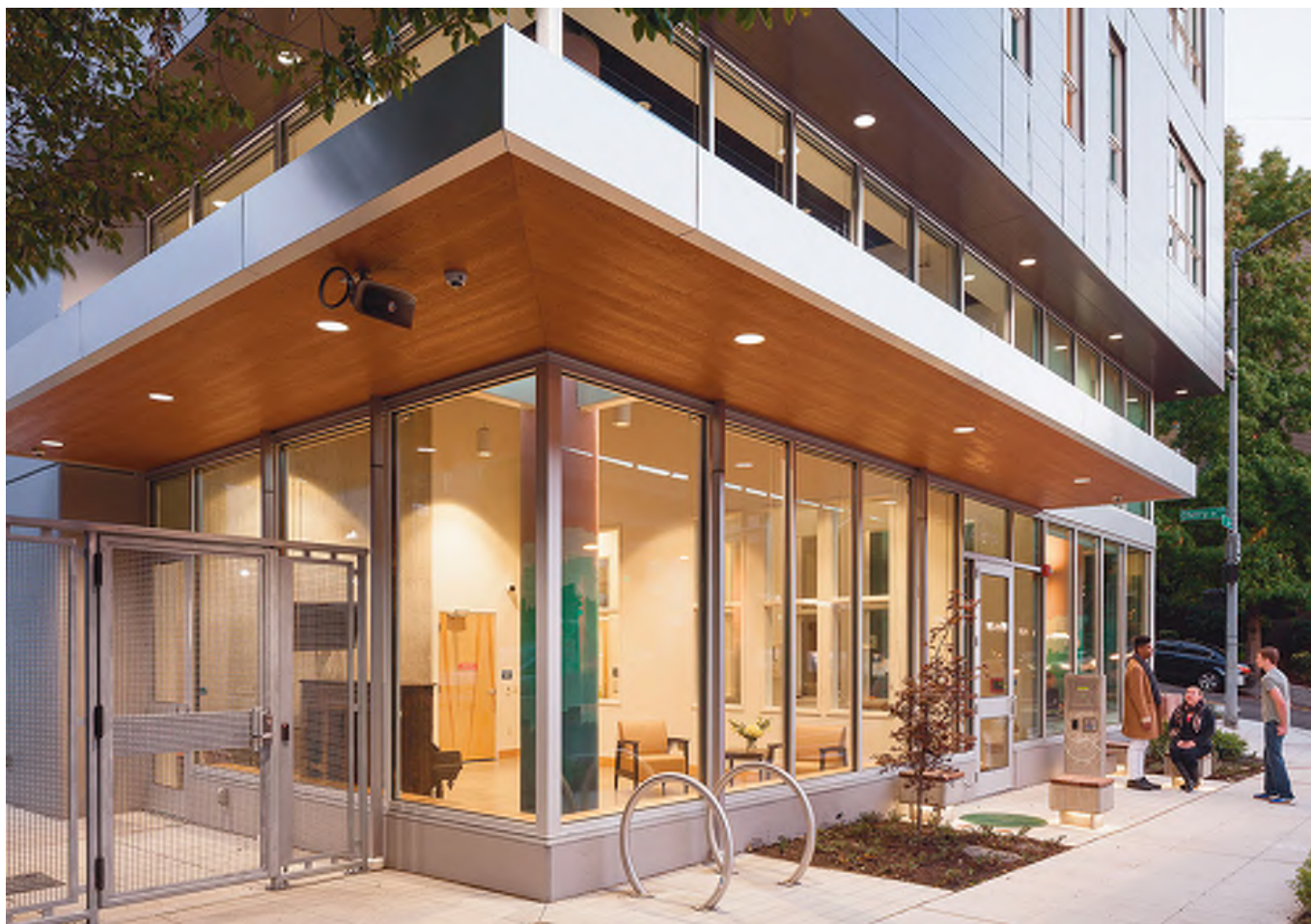
Carless in Seattle: Plymouth on First Hill's apartments are now home to some of the city's formerly homeless disabled population. Photo courtesy SMR Architects and Plymouth Housing Group.
