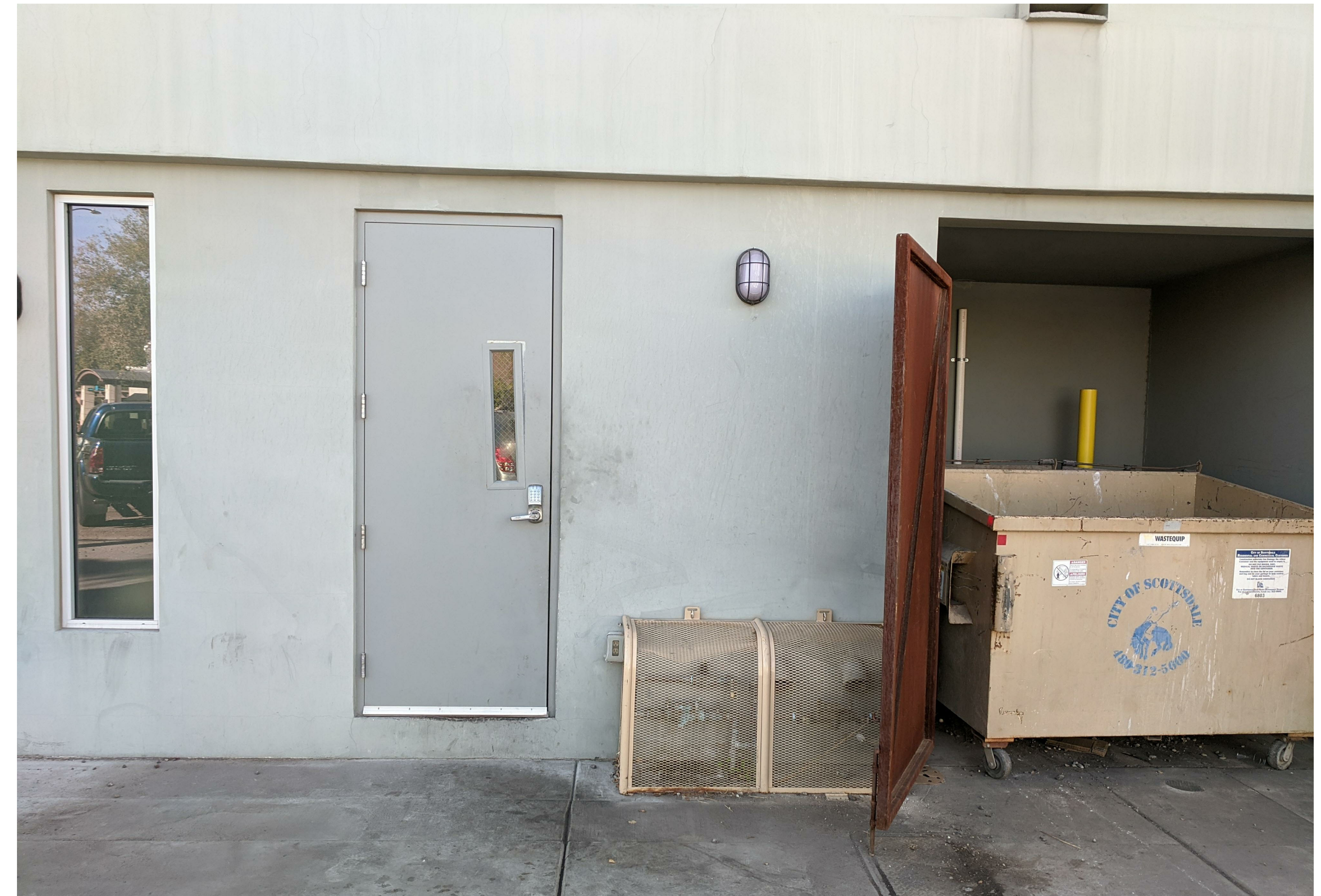
21 VIEW LOOKING TOWARDS THE SOUTH FROM THE ALLEY AT THE BACKSIDE OF THE ADJACENT EXISTING BUILDING
