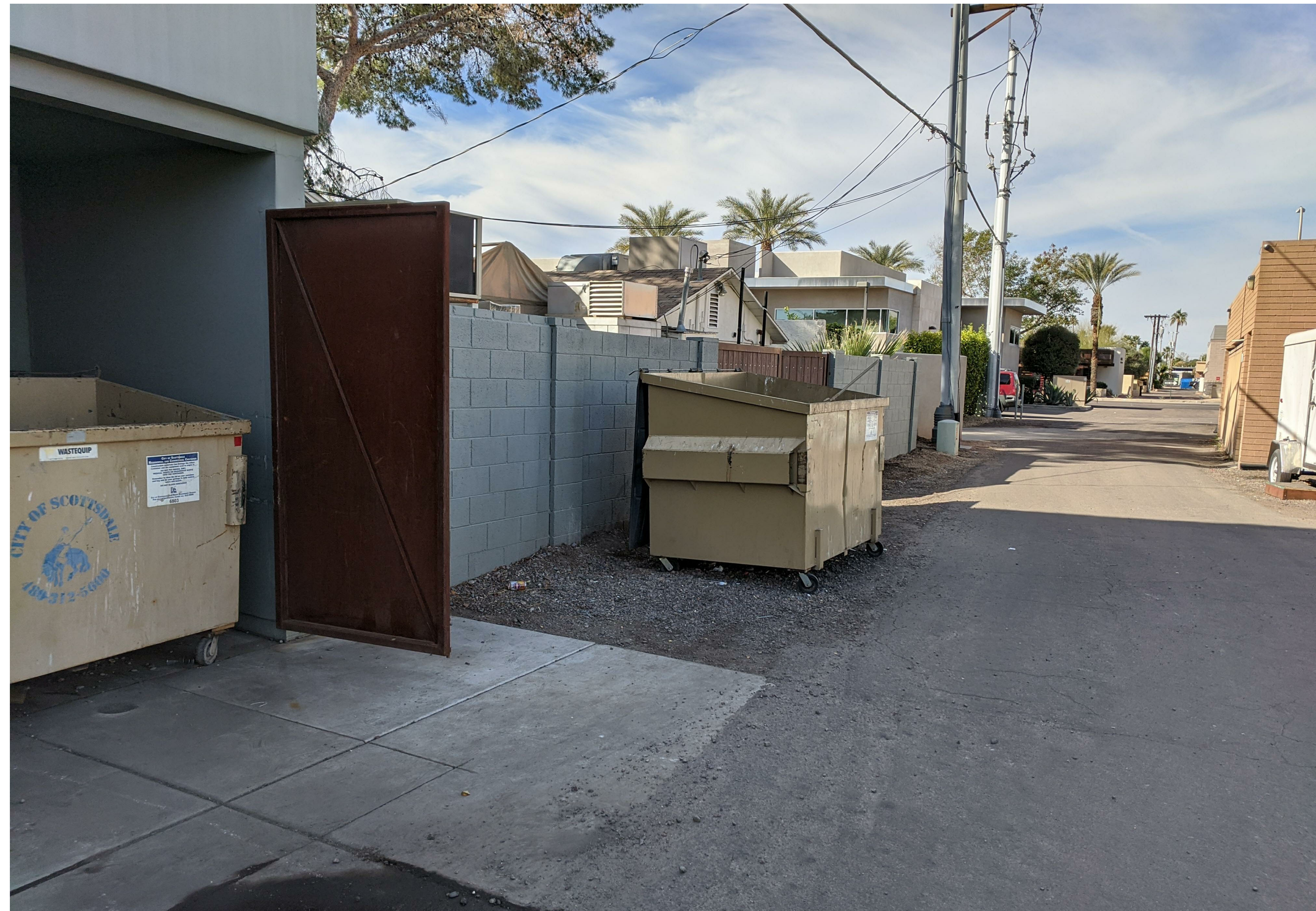
20 VIEW LOOKING TOWARDS THE SOUTHWEST/WEST FROM THE ALLEY OF THE EXISTING GARBAGE WASTE CONDITIONS
