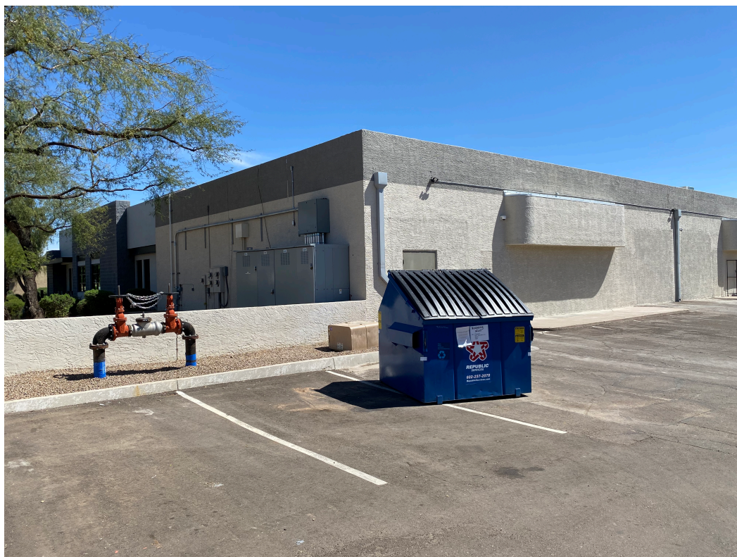
Picture 7: Sprinkler System Backflow Preventer
