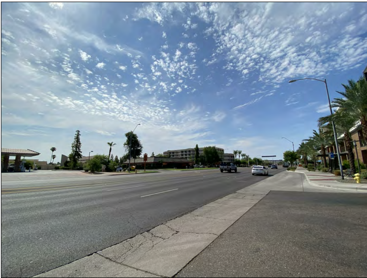
VIEW 11 From N. Scottsdale Rd. Looking SE
