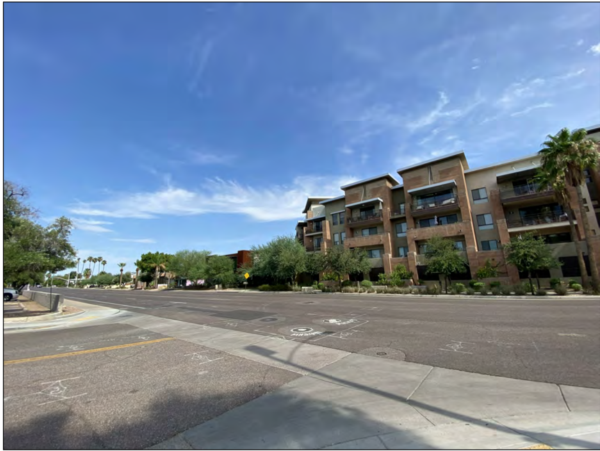
VIEW 4 From East Osborn Rd. Looking NW
