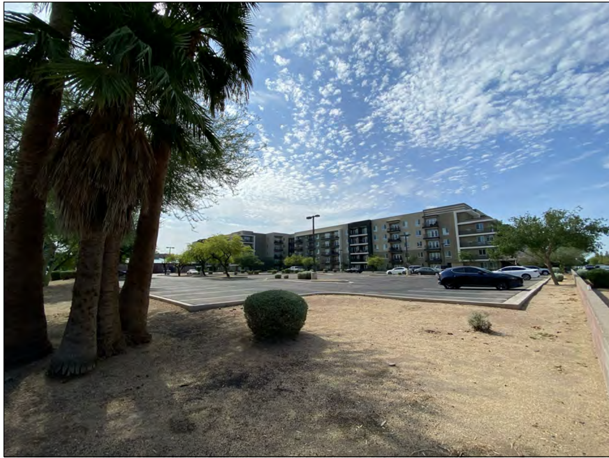
VIEW 2 From East Osborn Rd. Looking SE
