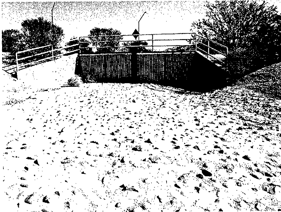
Photo 1: Downstream outlet from 10'x3' arch culvert.
