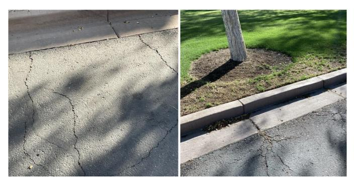
The retaining walls have been damaged by the roots of the Sissoo trees.
