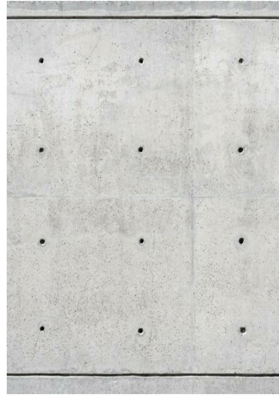
CONC-2 DESCRIPTION: CAST-IN-PLACE CONCRETE LOCATION: CAST-IN-PLACE CONCRETE WALLS COLOR: NATURAL GREY TEXTURE: SMOOTH (SNAP-TIE)
