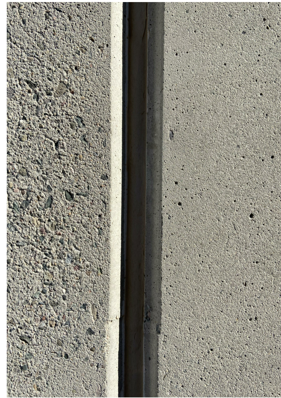
CONC-1 DESCRIPTION: SEALED CONCRETE LOCATION: TILT CONCRETE WALL PANELS COLOR: NATURAL GREY TEXTURE: SAND BLASTED
