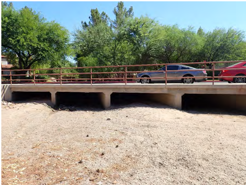
Photo 5: Looking South, downstream of Unnamed Wash. Four box culverts convey runoff under a private driveway. Note the sediment and debris collected in the culverts.
