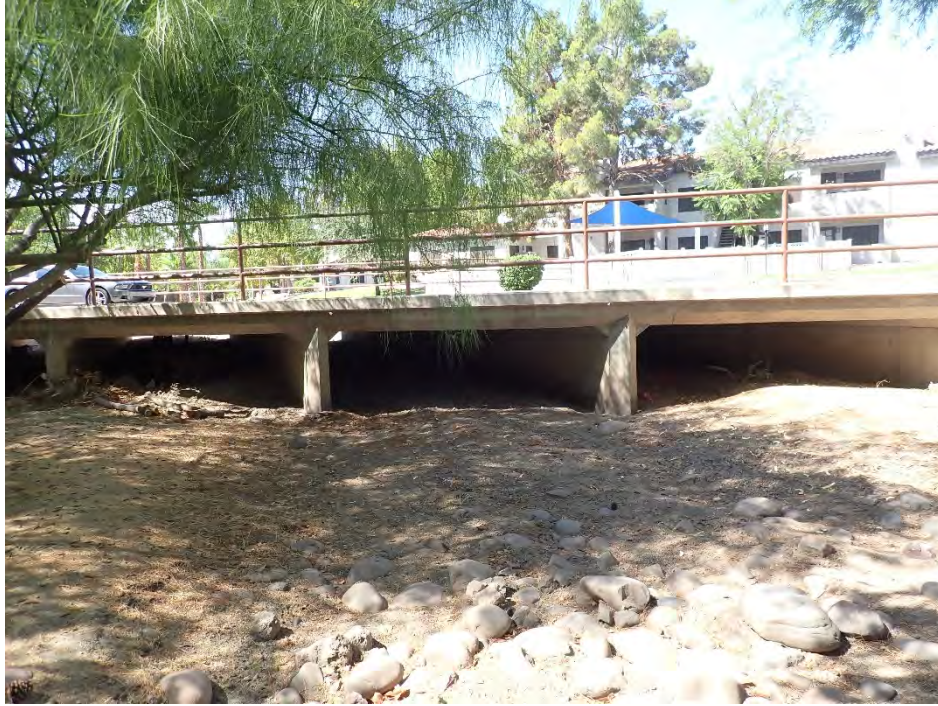
Photo 5: Looking South, downstream of Unnamed Wash. Four box culverts convey runoff under a private driveway. Note the sediment and debris collected in the culverts.
