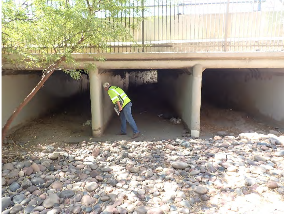
Photo 9: Looking South, downstream of Unnamed Wash. Three box culverts convey runoff under Mountain View Road.
