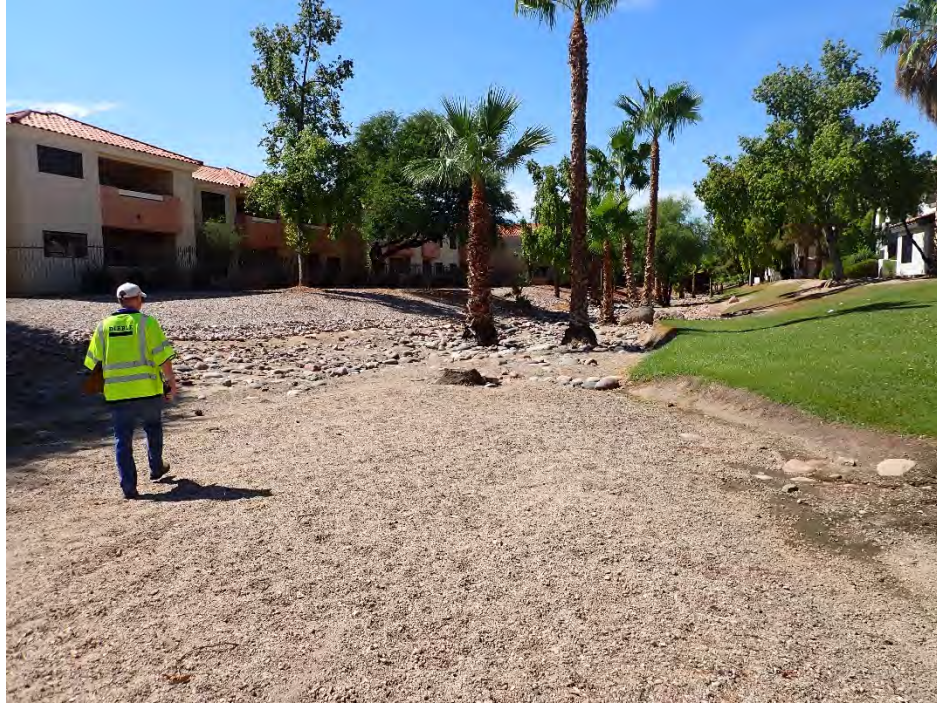
Photo 7: Looking South, downstream of Unnamed Wash. The banks are lined with gravel and grass. The main flow channel is gravel and has some vegetation obstructions.
