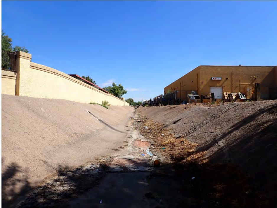
Photo 1: Looking North, upstream of Unnamed Wash. The channels material is shotcrete. Trash and other debris can be seen in the main channel.
