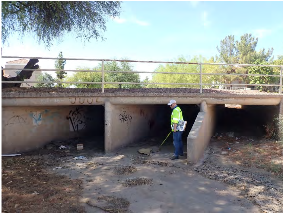
Photo 1: Looking North, upstream of Unnamed Wash. The channels material is shotcrete. Trash and other debris can be seen in the main channel.
