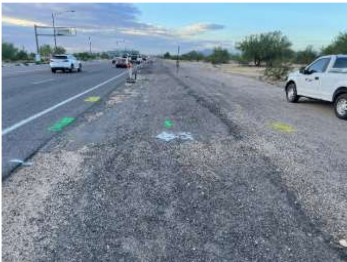
Figure 2.1.1 Shoulder and Utilities
