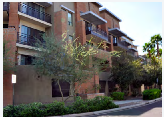
DISCOURAGED - Podium parking with no active uses at the street level.
