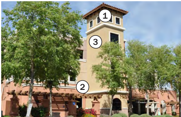
5th Avenue public parking garage.
