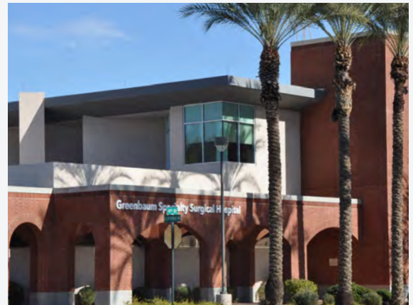
ENCOURAGED - Brick, the heaviest material within this building’s design palette, anchors the structure to the ground plane.
