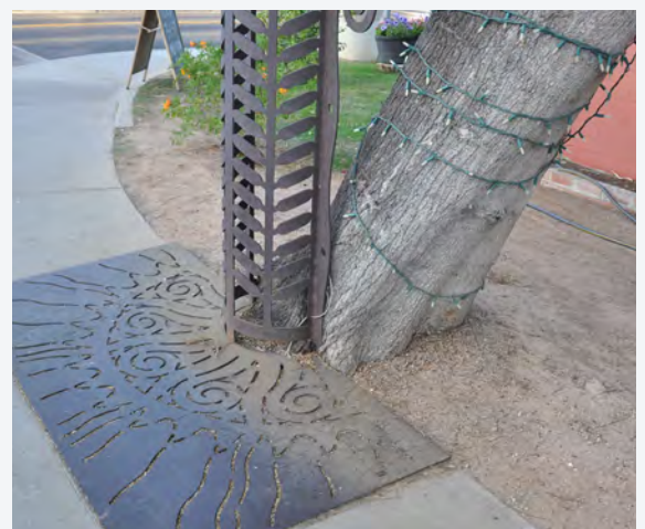
Landscape planting can damage sidewalks, building foundations, and utilities if not located appropriately to allow for mature growth and maintenance needs.
