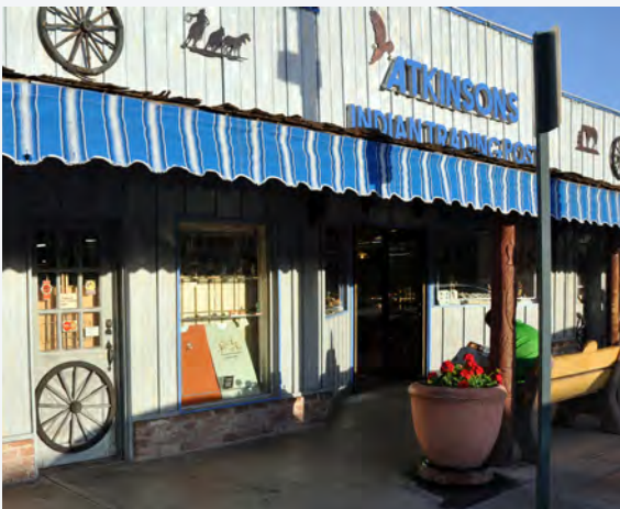
This storefront incorporates a traditional style covered walkway, wood-frame windows, and a brick wainscot below board and batten siding. The storefront has multiple entrances and doorways that are recessed as well as decorative, Western details.
