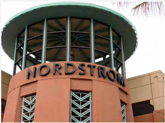
The corner of this parking garage is articulated as a stair tower giving the structure the appearance of a building.
