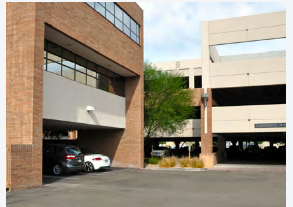
A single parking bay incorporated into the building design, and internal to the site, beneath the second floor.
