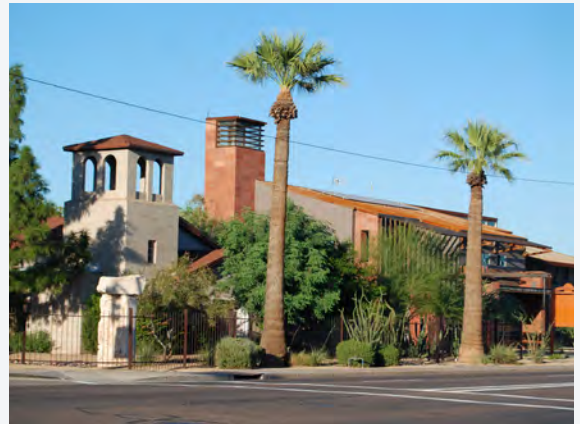
The balance between the new building design of the fire station with the existing church design (foreground) is strengthened by shared features such as concrete block as a key material, tower and roof features with similar geometry, similar roof pitch, street continuity, and metal picket fencing.
