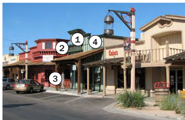
Old Town street frontage.
