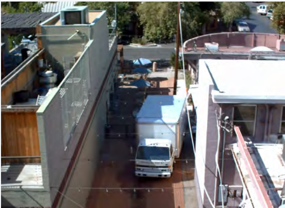
Alley service/deliveries and screened building equipment are encouraged.
