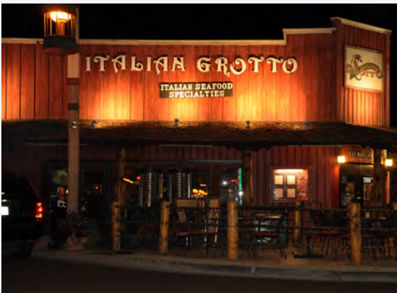
This sign represents cut-out letters applied to the painted wall surface, indirectly illuminated.
