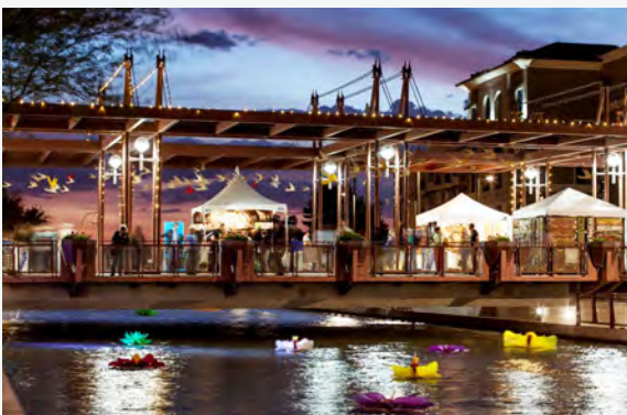
Incorporation of permanent infrastructure, such as the Marshall Way Bridge, in open spaces supports day-to-day activities and events year-round.
