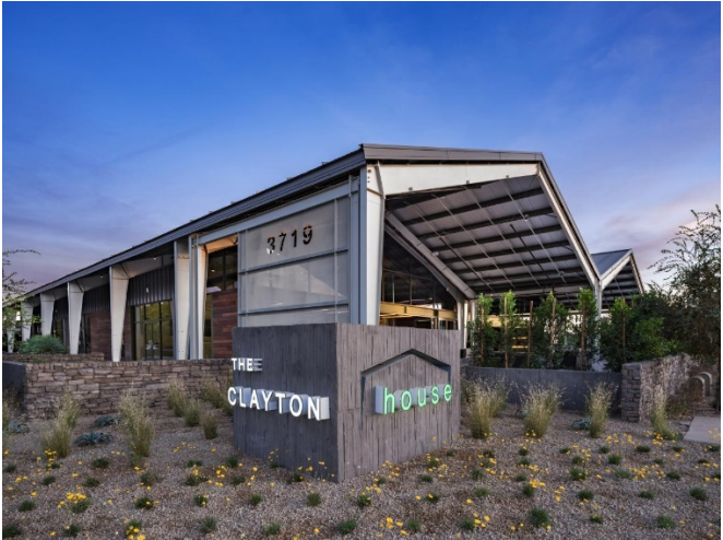
The CLAYTON House SEC of 75 th & 2 nd St
