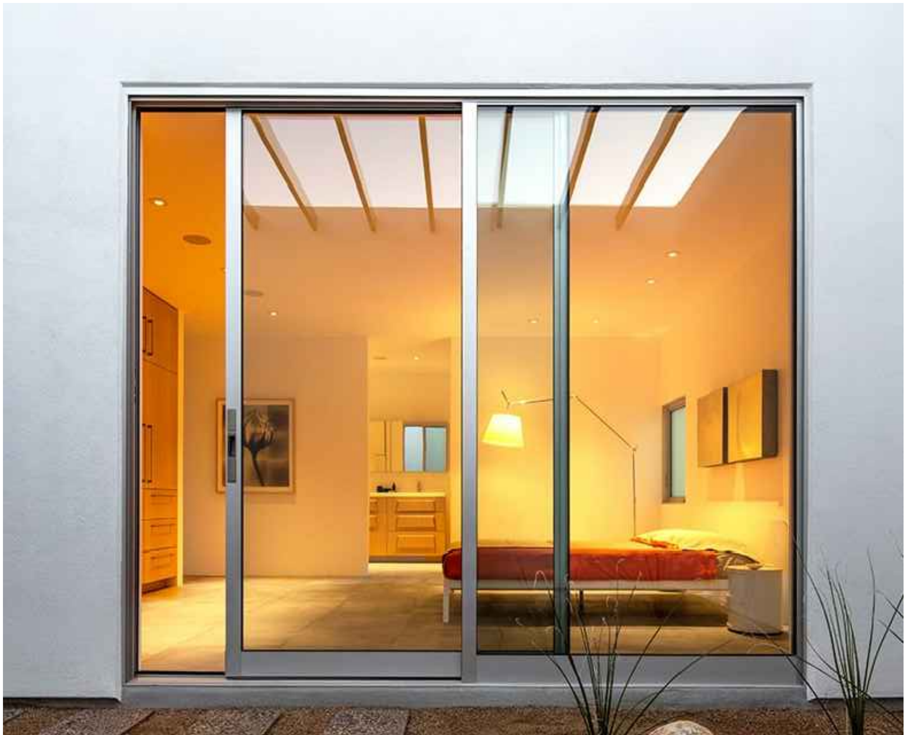
[WIN-1] CLEAR ANODIZED THERMALLY BROKEN ALUMINUM WINDOW/DOOR FRAME W/ 1" INSULATED GLAZING WITH LOW-E COATING
