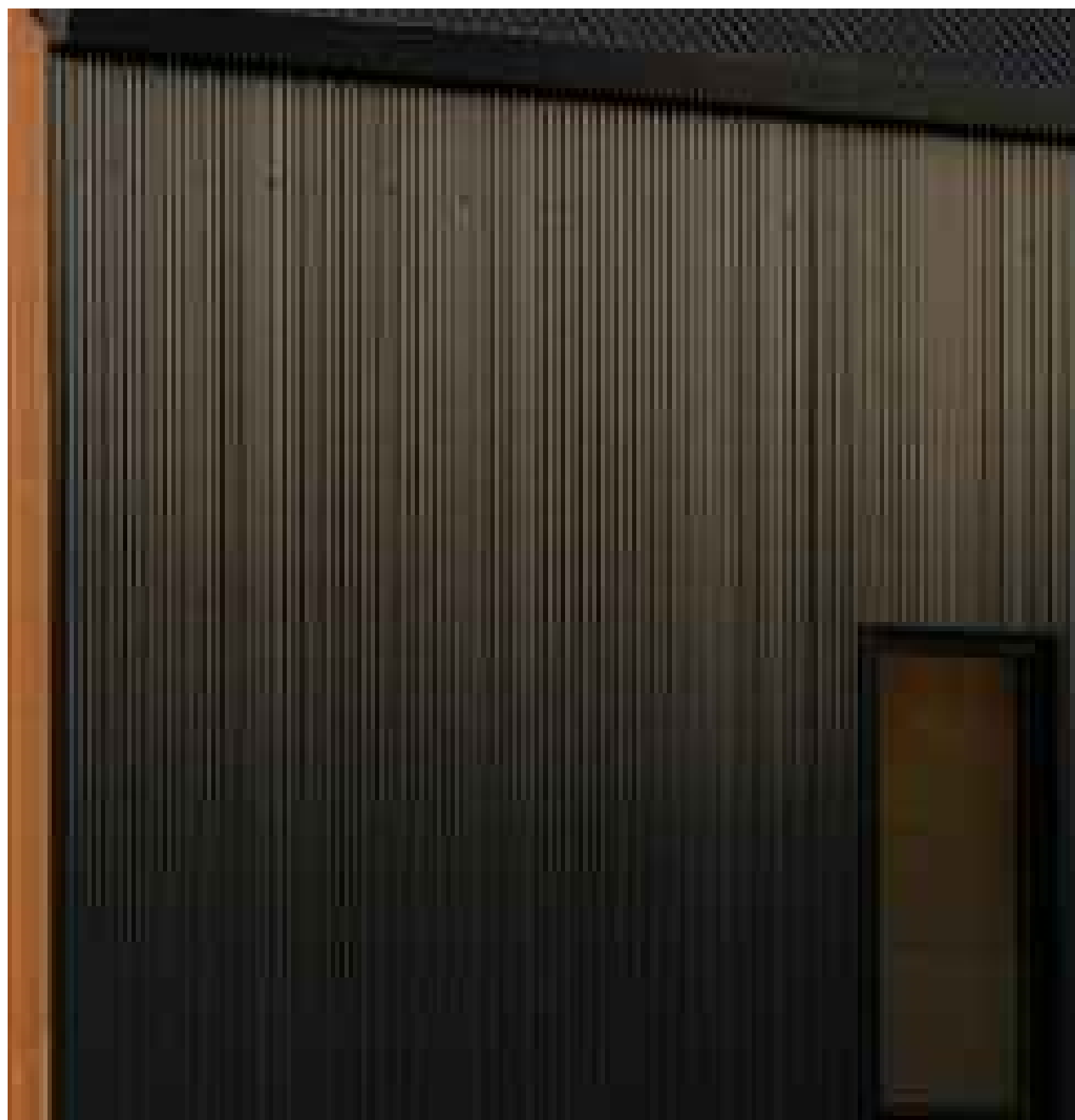
[MTL-2] 22GA 7/8" CORRUGATED METAL WALL CLADDING W/ BRONZE ANODIZED FINISH
