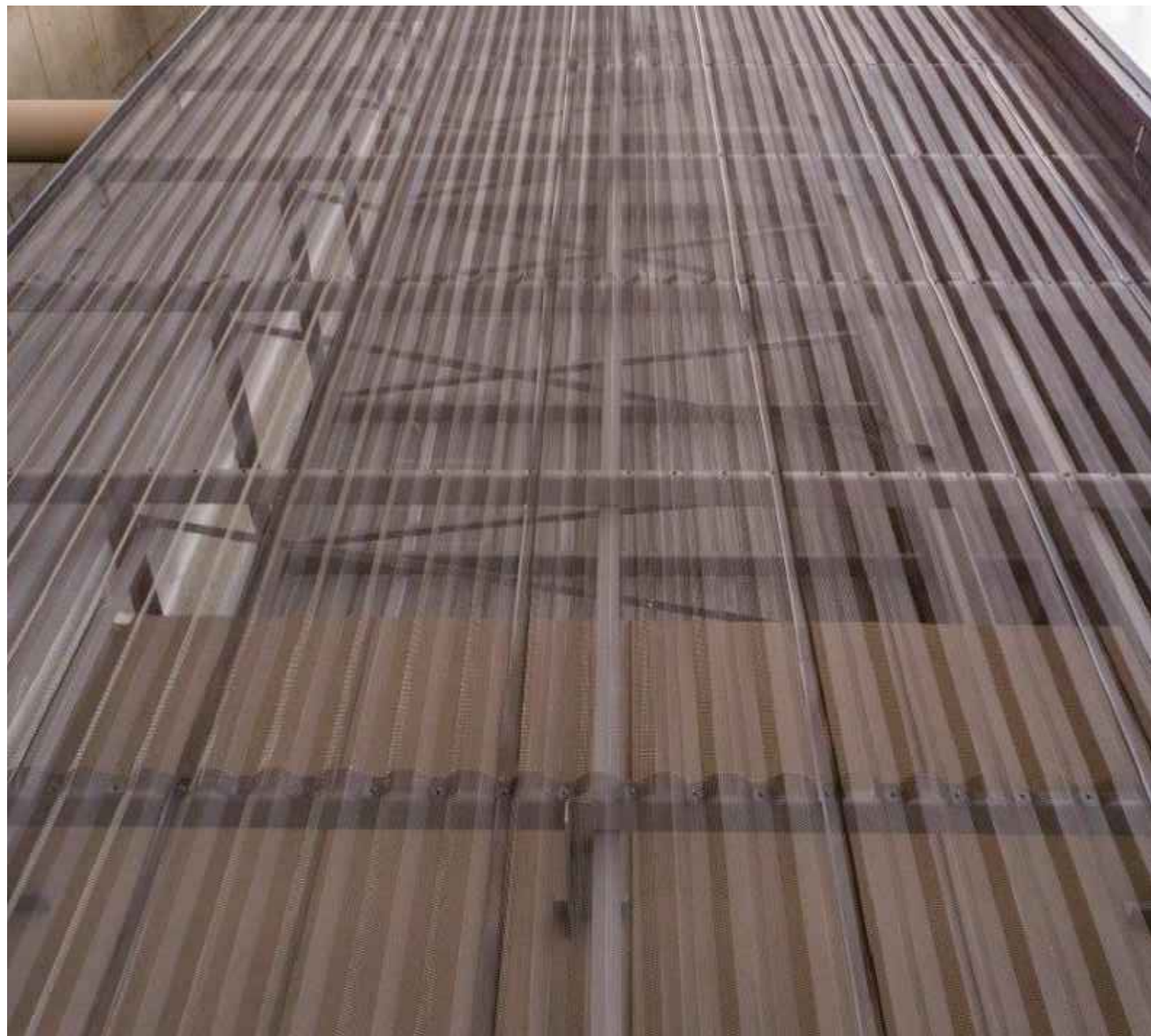
[MTL-3] PERFORATED 22GA 7/8" CORRUGATED METAL WALL CLADDING W/ BRONZE ANODIZED FINISH
