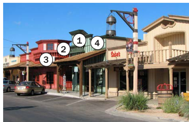
Old Town street frontage.
