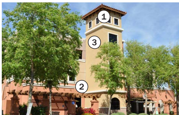
5th Avenue public parking garage.
