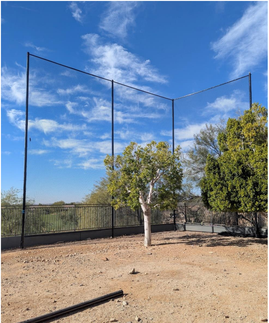
Initial installation – 30 feet
