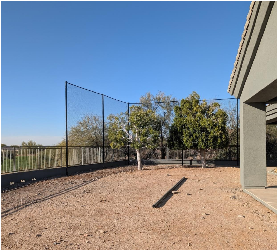
Current installation – 20 feet
