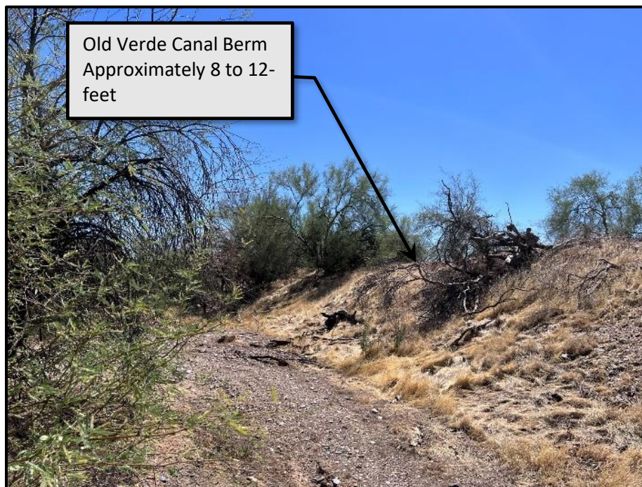
Figure 2: Existing Old Verde Canal Berm
