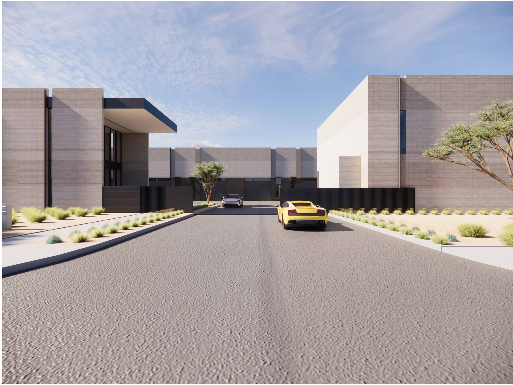
NORTH VIEW - MAIN GATE
