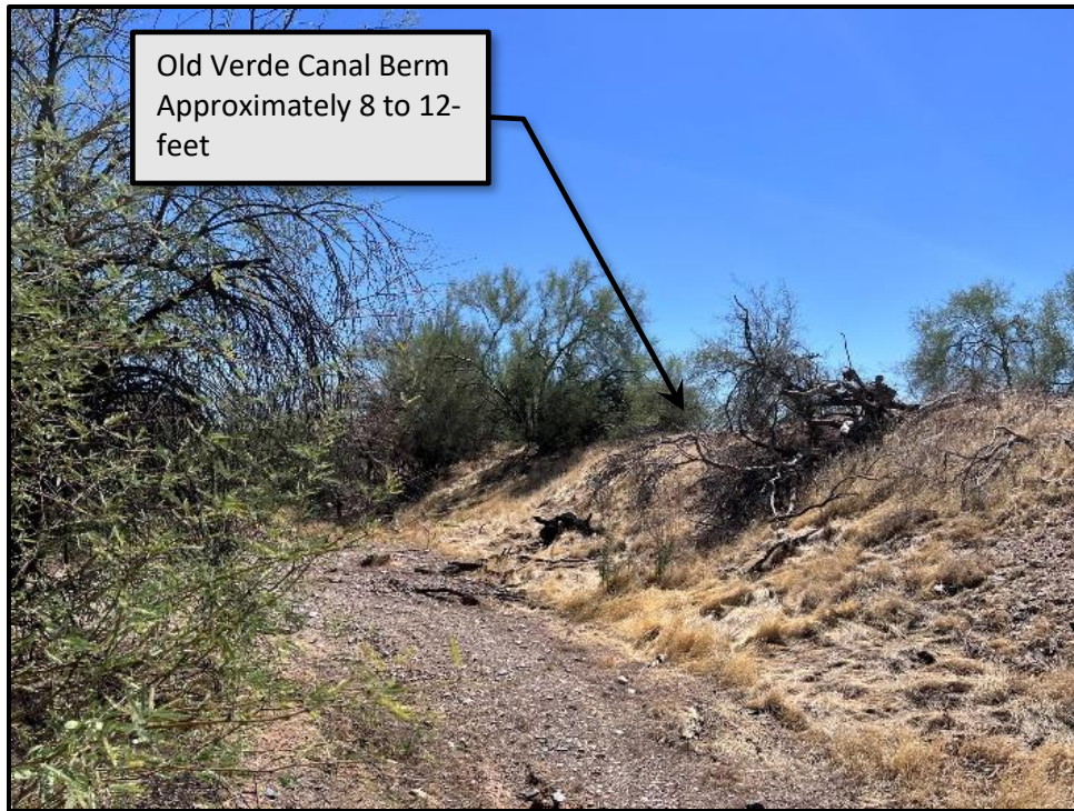
Figure 2: Existing Old Verde Canal Berm
