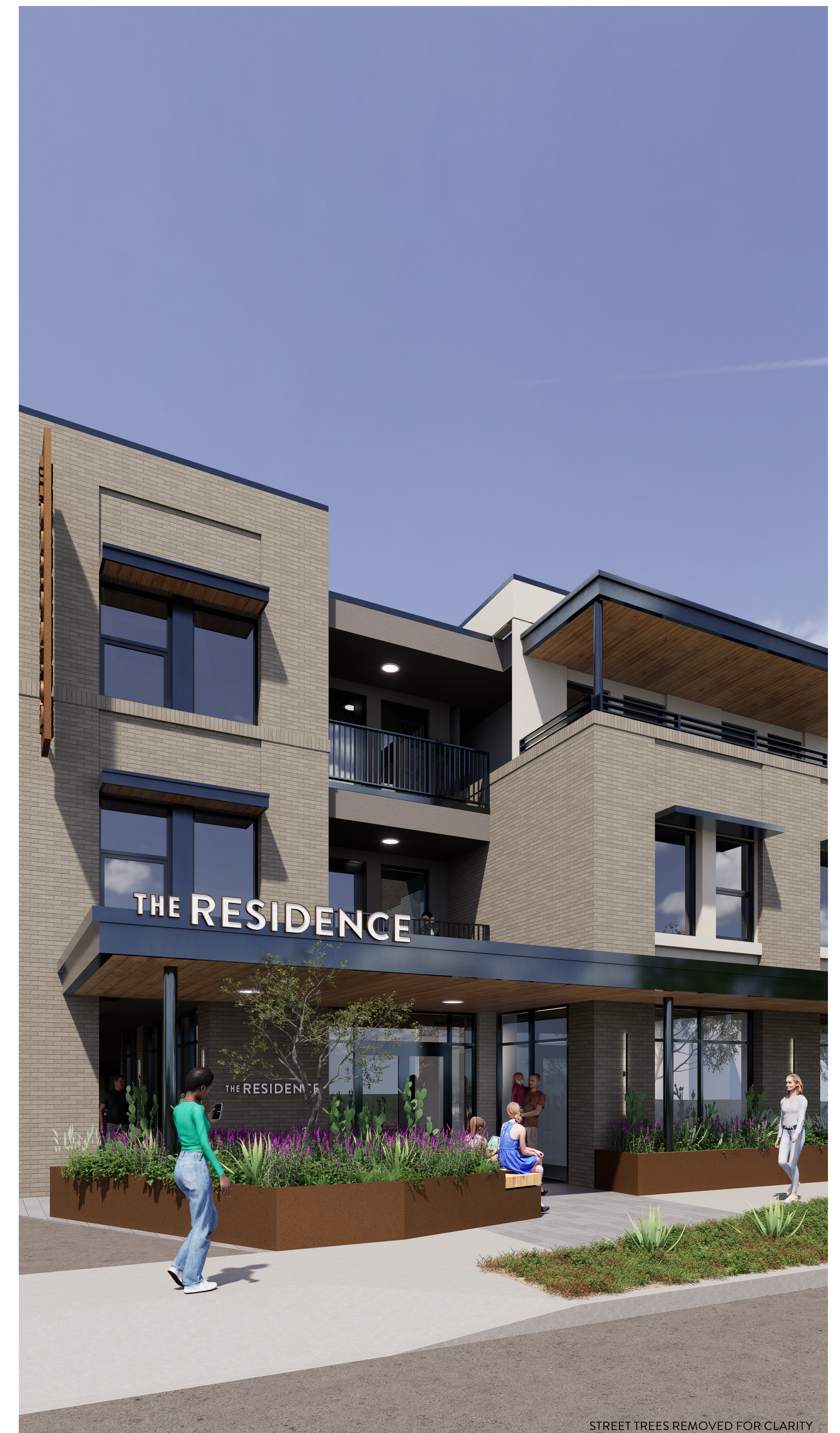
MAIN ENTRY ON N. MILLER ROAD
